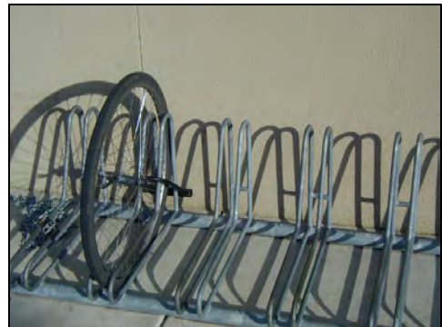
Bad bicycle racks can complicate locking the bicycle, make theft easy or cause a wheel to be bent.
