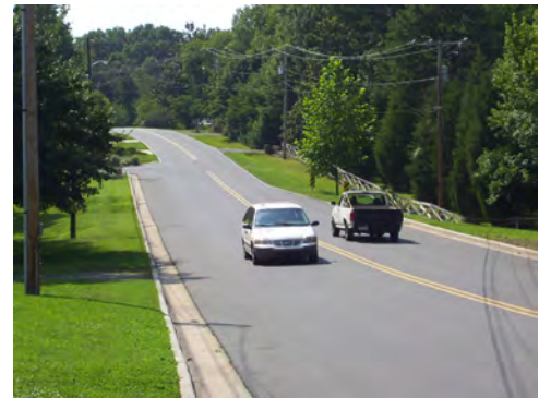
This portion of Park Ridge Road is over 40 feet wide from curb to curb, suitable for striped bicycle lanes.
