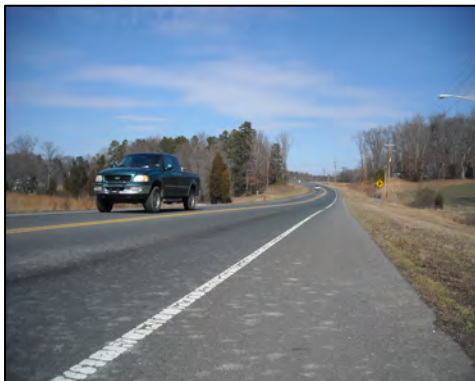
This photo was taken on the Northeast Connector in Albemarle. This shoulder is approximately 3 feet wide, but a minimum of 5 feet is preferred.
