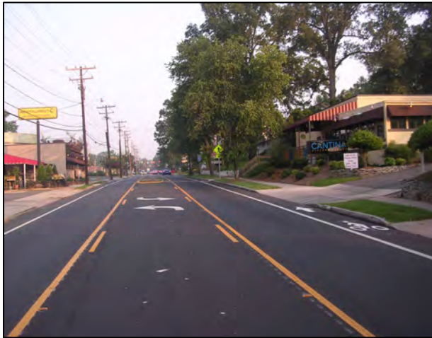
A road diet created bike lanes and a new center turn lane on a former 4-lane undivided roadway in Charlotte.
