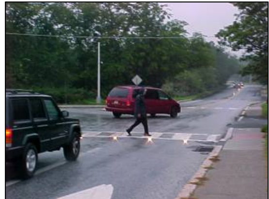
In-pavement flashing crosswalks improve visibility
