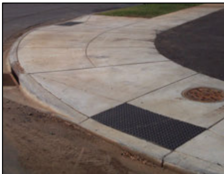
New sidewalks with ADA considerations.
