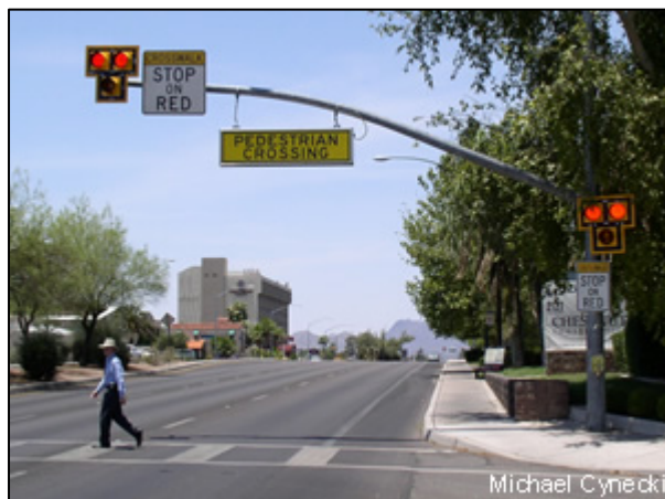
A HAWK signal in Tucson, Arizona
