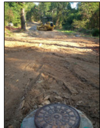
Sewer lines near Summit
