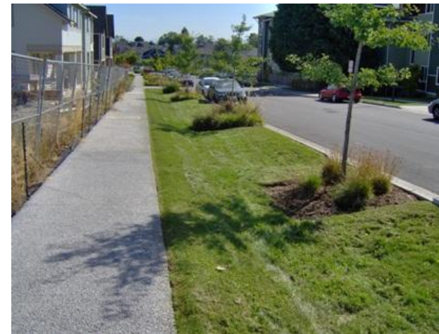
Figure 4-15. Top: Vegetated swale and porous concrete sidewalk help to make a “green street” in the new urbanist development of High Point in West Seattle. Right: Porous asphalt allows the passage of water through small openings, or pores, that are atypical of standard asphalt. Source: Rhode Island Cooperative Extension
