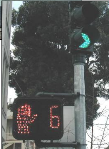
Figure 4-6. Countdown pedestrian signals indicate to pedestrians how much time is left to safely cross the street before the close of the traffic cycle.
