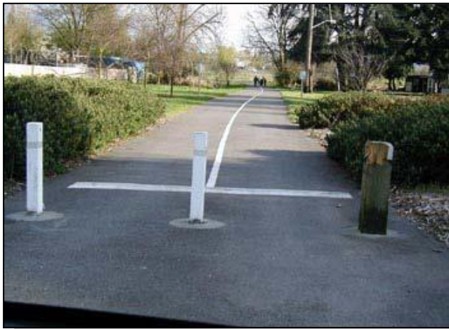
Figure 4-14. Typical greenway cross-section with bollard treatments at roadway crossing.
