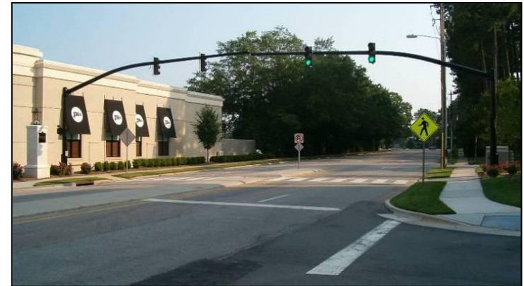
Figure 4-7. Examples of pedestrian- activated, signalized, mid-block crossings.
