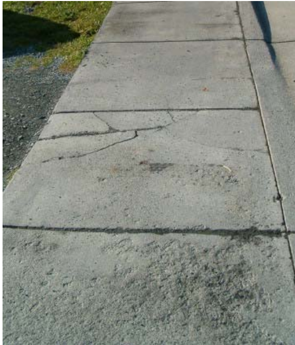
Figure 5-5. Greenway & Sidewalk Maintenance. While many of Banner Elk's sidewalks and trails are new and therefore in good repair, both will eventually need repair for cracking (below sidewalk on Main Street), overgrowth, debris removal, or undercutting caused by runoff (see Town Park Trail below).
