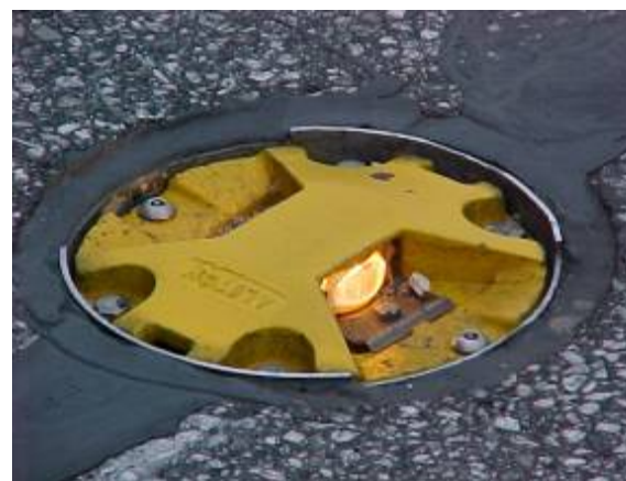
In-pavement flashing warning light system
