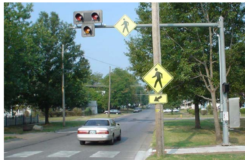
Pedestrian activated warning signals with signage at a midblock crosswalk
