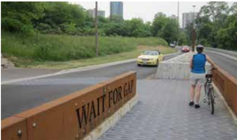
A z-crossing of a greenway through a major road prioritizes the safety of all users. Signals may be added.
