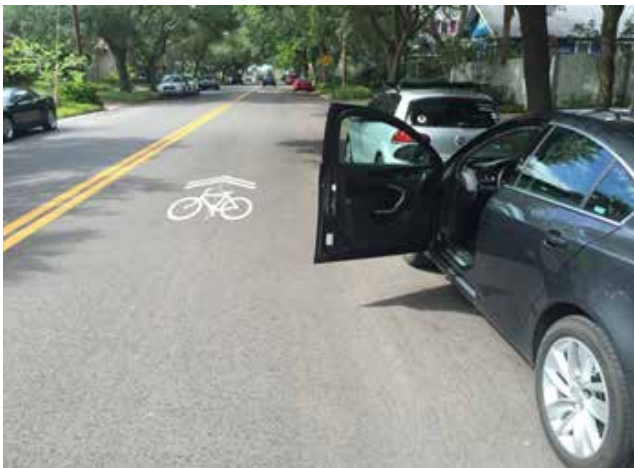
Placing sharrows outside the “door zone” is important in areas with on-street parking.
