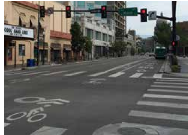
Sharrows can also be used to guide bicyclists in shared lanes through intersections to bike lanes.
