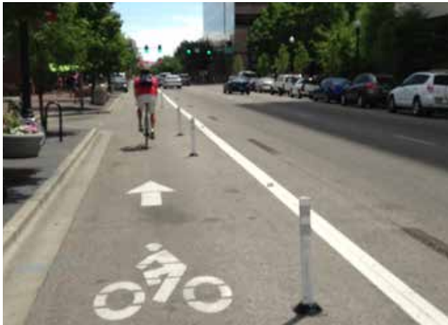
A simple cycletrack can integrate plastic “candlesticks” to better delineate space on the street.
