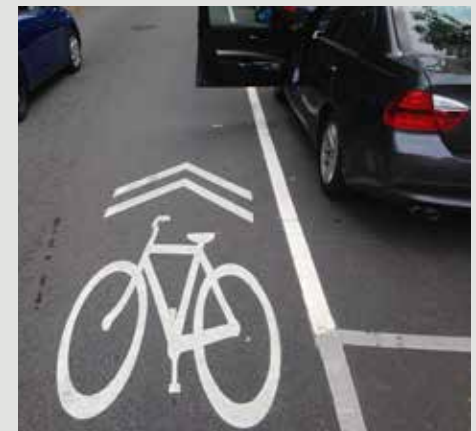
Shared lane marking
