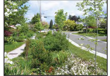
Figure 6(x): Landscaping used on the Sea Street in Seattle, Washington shows how stormwater treatment can be tied to aesthetically pleasing plantings 7 .
