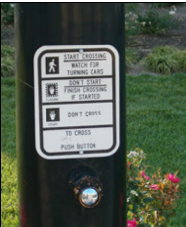
Figure 5-5. Examples of pedestrian-activated signalized mid-block crossings. Top image: An example of a pedestrian-activated signalized mid-block crossing. Bottom image: An at-site guide for pedestrians to assist them in understanding the meaning of the push-button signals.
