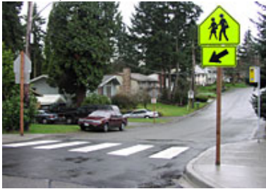
Fig. 5-4: Bulb-outs create a shorter crossing for the pedestrian and make them more visible to drivers around parked cars. This is a mid-block crossing utilizing a high-visibility crosswalk.
