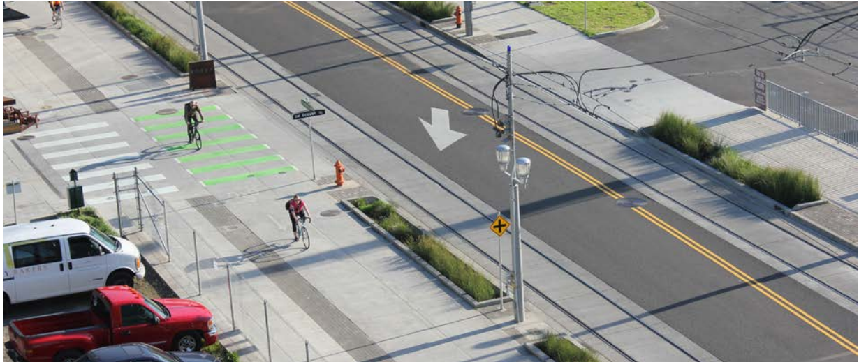
Intersection crossing markings can be used at signalized intersections or high volume minor street and driveway crossings, as illustrated above.
