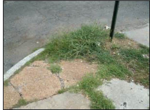
Broken, overgrown sidewalks are not ADA compliant
