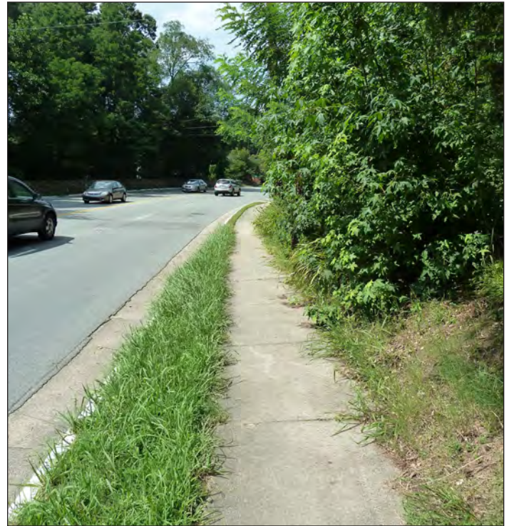
ABOVE: Along with deteriorating and broken sections of concrete, encroaching vegetation can limit the usable space of sidewalks significantly.
