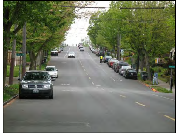
Climbing lanes include a five-foot bicycle lane on one side of the roadway and a shared lane marking on the other side of the roadway.
