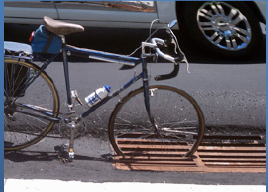
Dangerous Drainage Grate for Bicycles
