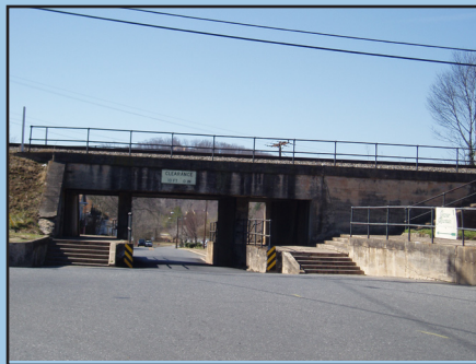
Rail underpasses do not meet ADA compliance and do not allow for proper visibility.
