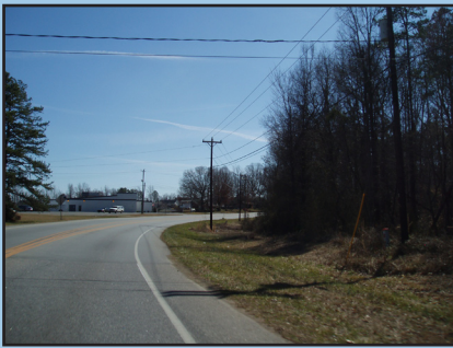
New Hope Road lacks curb and gutter and pedestrian facilities such as sidewalks and crosswalks.
