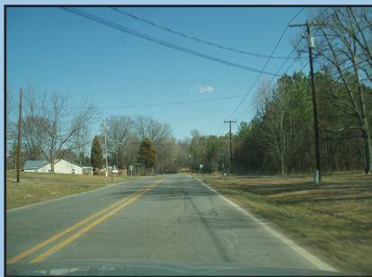
Armstrong Ford Road lacks curb and gutter and has no pedestrian facilities such as sidewalks and crosswalks.
