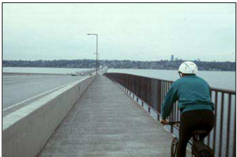
Metal railing and a concrete barrier wall provide a safe and functional area for pedestrians and bicyclists.
