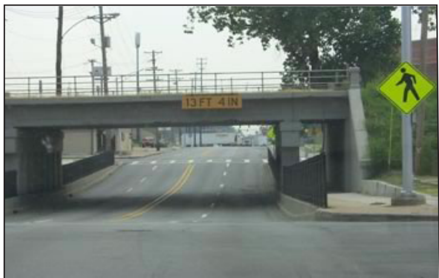
Pedestrian underpass with metal railing for pedestrian safety and separation. Photo credit: ITE Pedestrian Bicycle Council
