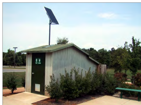
A solar-powered rest room
