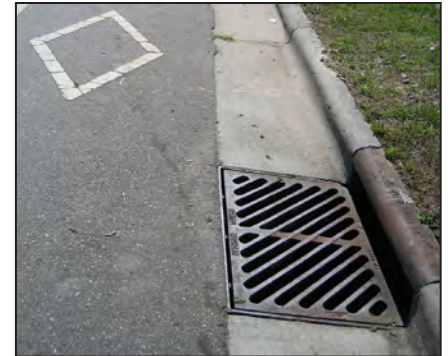
Bicycle-Friendly Drainage Grate
