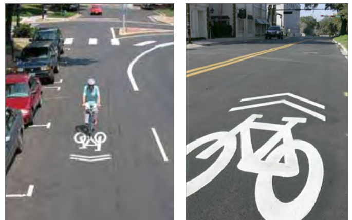
Sharrows installed on lanes that are too narrow for striping designated bike lanes.
