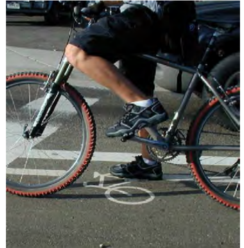
Above: Add bicycle-sensitive loop detectors and use pavement marking to aid bicyclists in locating them at intersections; see Chapter 4: Bicycle Facility Standards for more information.
