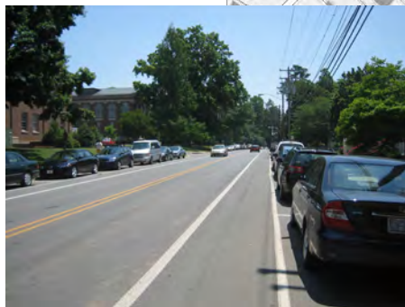
Above: Existing bike lanes on Concord do not provide enough room for cyclists to avoid the 'door zone' of parked cars.
