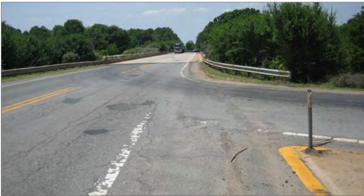
Example Project: Sidepath across I-77 Bridge and exit ramps (see draft plan pages 39 and 101, for all project recommendations).
