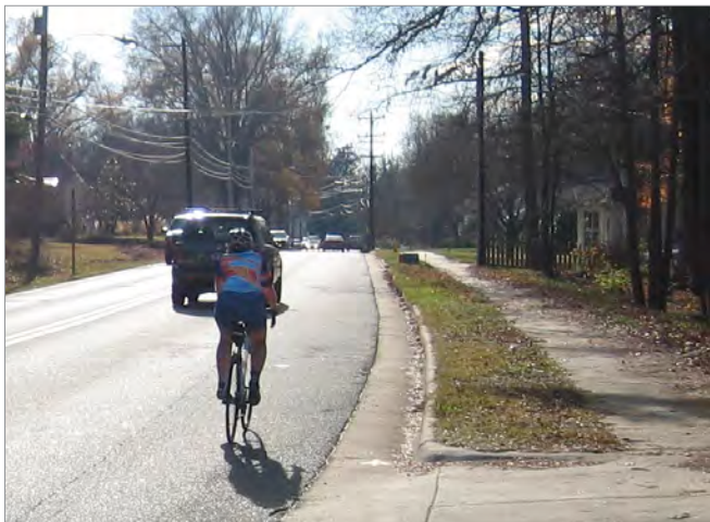
Above: Existing conditions on N Main Street will allow for a simple restriping of the roadway to allow bicycle lanes.
