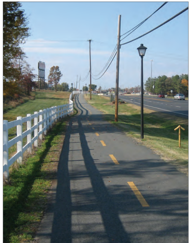
Sidepath example without curb and gutter in Conover, NC.
