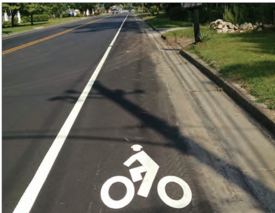
Above: During this planning process, King Street was resurfaced and bicycle lanes were added to provide safe access for bicyclists to Town parks and other destinations.
