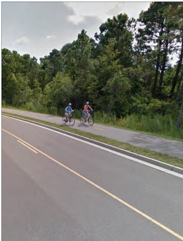
Sidepath example with curb and gutter in Wilmington, NC, along Museum Dr.
