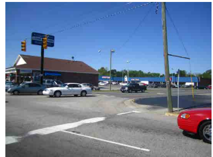
Sidewalks along Poplar Street have unsafe crossings and numerous driveway cuts.
