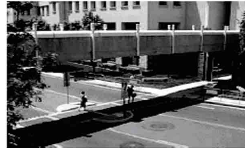
Pedestrian bridges can be problematic in that they are expensive and sometimes pedestrians don't use them ; Source: DBPT
