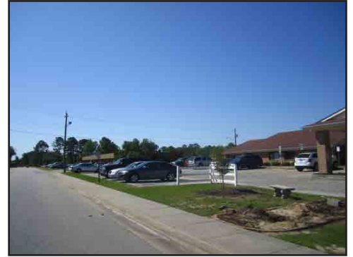
The existing sidewalks on Mercer Road are narrow and should be a minimum of 5 feet wide.
