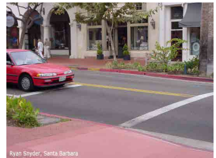
Advance stop bar at a crosswalk; Source:caactive-communities.org
