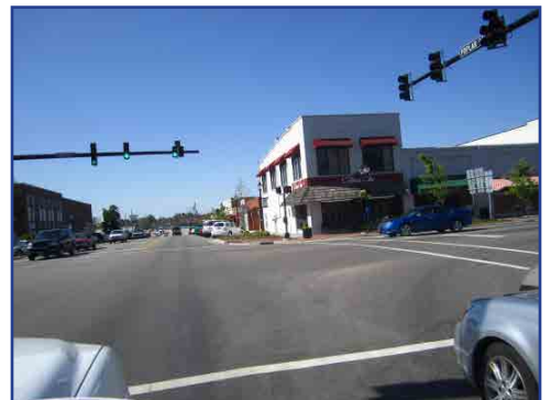
The crosswalks on Poplar Street at Broad Street would benefit from enhancements calling motorists’ attention to this heavy pedestrian area.
