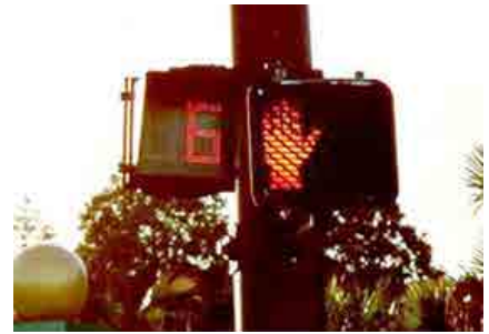
International symbol for a pedestrian crossing, along with a countdown signal; Source: ITE Pedestrian Bike Council
