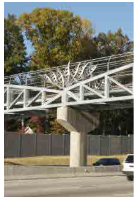
Pedestrian bridges, such as this one in Cary, NC, can provide connectivity and opportunities for art
