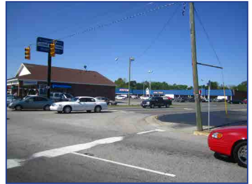
The intersection of Swanzy and Poplar Streets needs a marked crosswalk and pedestrian signalization.
