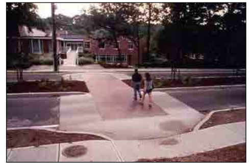
Raised Crosswalk; Source: DBPT
