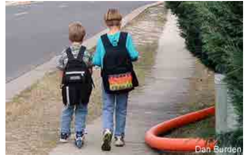
This four-foot wide sidewalk is too narrow for comfortable walking and navigating possible obstacles. Source: Safe Routes to School
