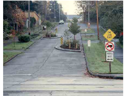
One-lane chicane slows down traffic; Source:Richard Drdul
