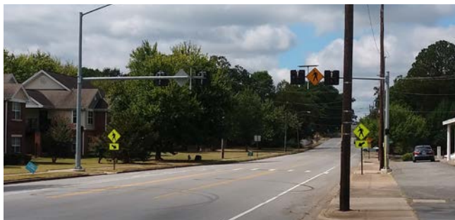
Pedestrian Hybrid Beacons stop automobile traffic for bicyclists and pedestrians wishing to cross a high traffic volume/high speed roadway.
