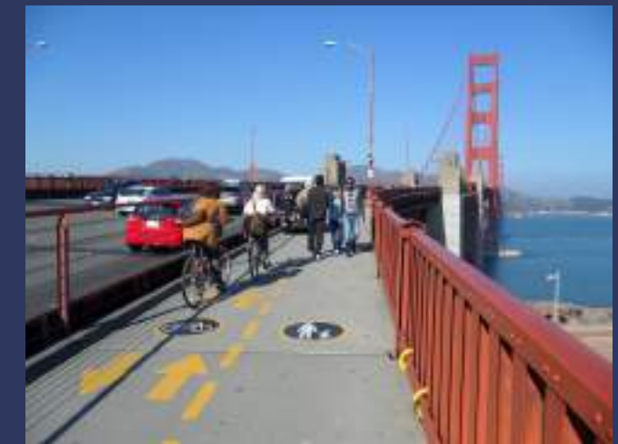
San Francisco, CA Golden Gate Bridge Pedestrian Crossing
