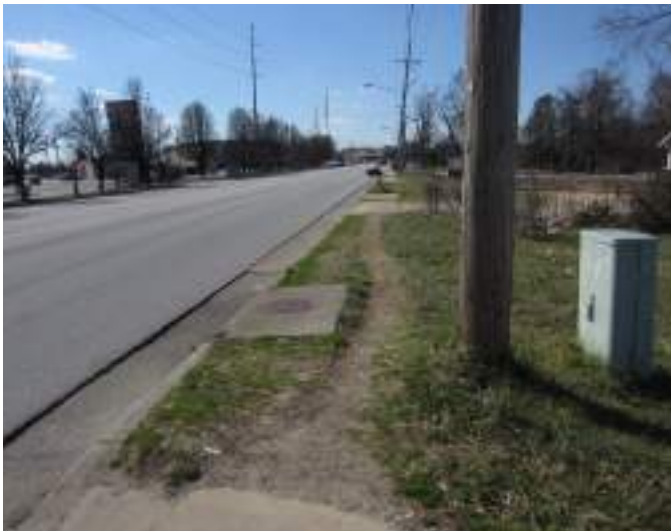
Worn foot path on Fairfield Road
