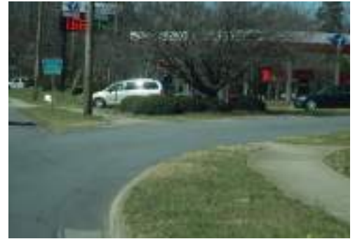
Lack of crosswalk at the I-85 ramp on Main Street
