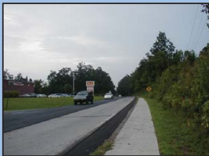
Inadequate Separation Between Pedestrians and Vehicular Traffic Makes for Hazardous Conditions.
