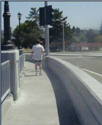
Pedestrian sidewalk on bridge with separation.
