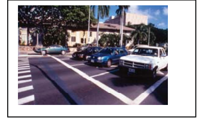
Advance stop bar Source: Pedestrian and Bicycle Information Center Image Library
