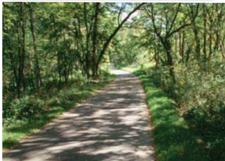
Greenway paths should be minimum 10' wide to accommodate both Pedestrians and Bicyclists
