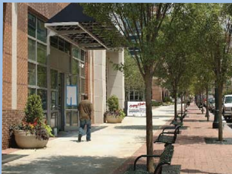
Buffer paving option and Tree Pits Photo credit: www.gatech.edu
