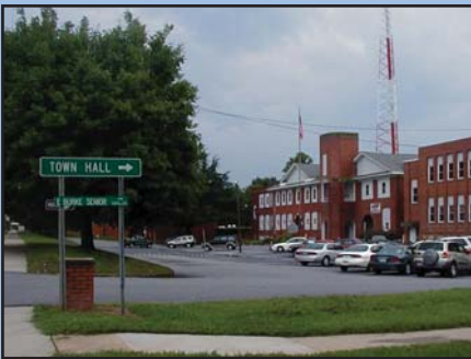
Pedestrian Facilities at Hildebran Town Hall
