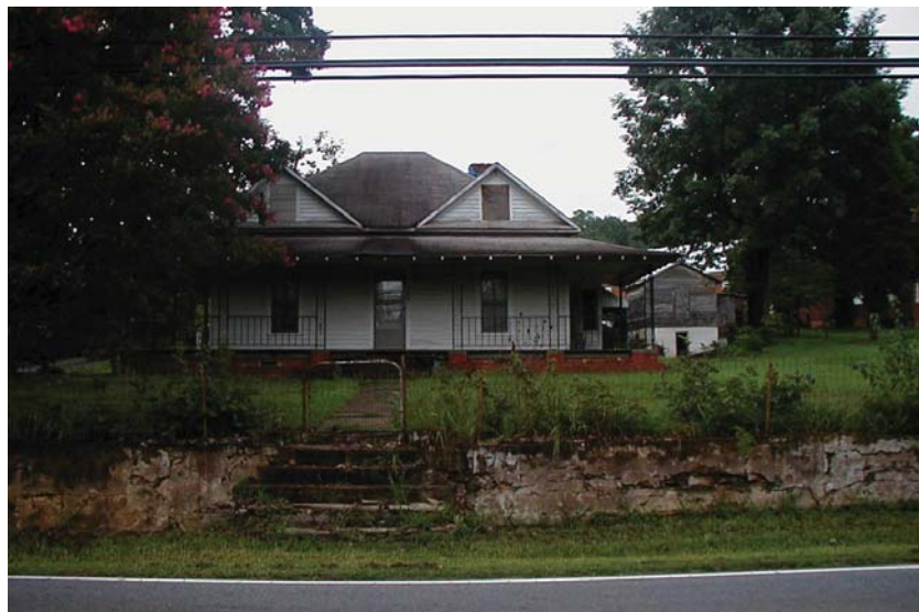
Lack of Pedestrian Facilities in Residential Neighborhood
