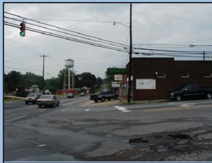
The absence of sidewalks along this Commercial strip on Hwy 70 creates dangerous conditions for Pedestrians
