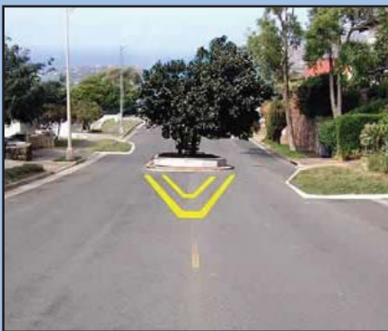
Chicane with a center island and curb extensions Photo credit: Dan Burden
