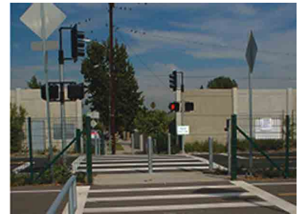
A "Z" type pedestrian crossing at a railroad, along with fencing to keep pedestrians on the sidewalk helps to increase safety and awareness at the crossing. Above diagram source FHWA.dot.gov
