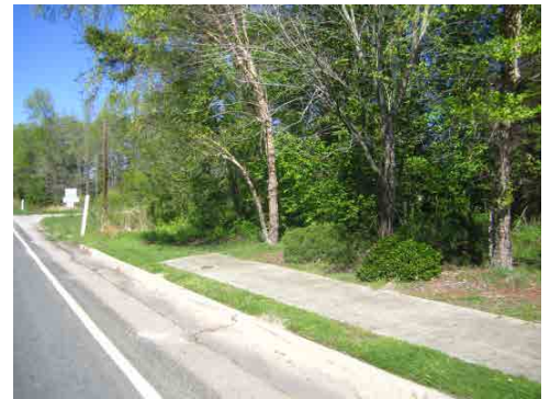
A small segment of sidewalk on Old Knight Road north of Knightdale Boulevard ends abruptly with no continuation
