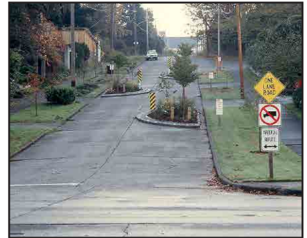
One-lane chicane slows down traffic; Source:Richard Drdul
