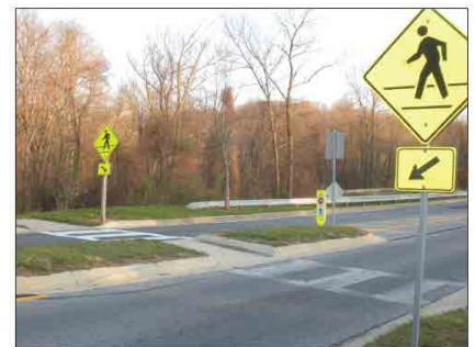
Mid-block crossing with pedestrian refuge island and signage; Source: fhwa.dot.gov
