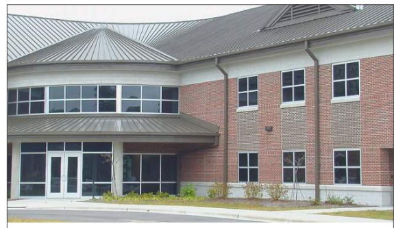
The new Leland Town Hall opened in 2015.
