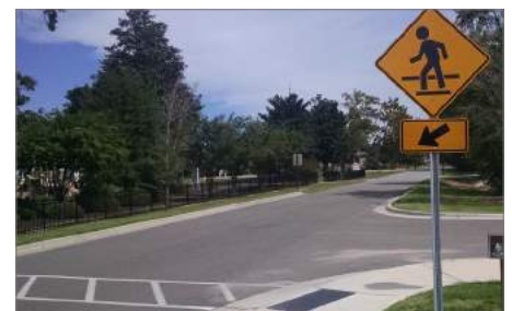
Pedestrian crossing with crosswalk, curb ramp, and signage (at Town Hall Dr).
