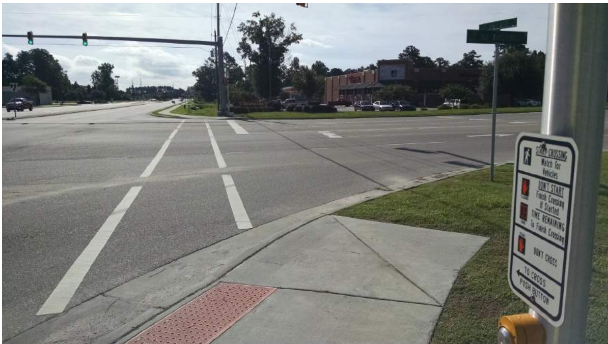
Village Road and Old Fayetteville Road intersection, which was recently improved with pedestrian amenities, including pedestrian countdown timers, marked crosswalks, and curb ramps
