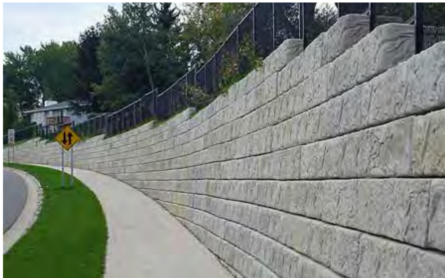
Pre-Cast Segmental Gravity Retaining Wall
