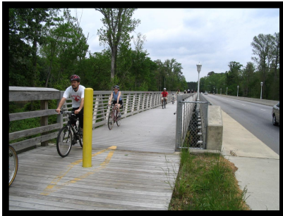
Cantilevered multi-use path
