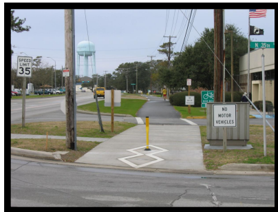
Bridges Street Multi-Use Path
