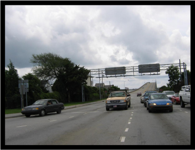
Atlantic Beach Bridge
