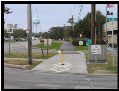
Bridges Street Multi-Use Path
