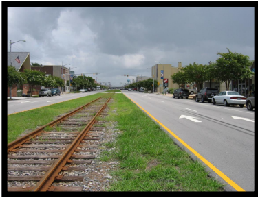
Arendell Street “Before”
