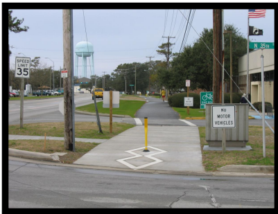
Bridges Street multi-use path
