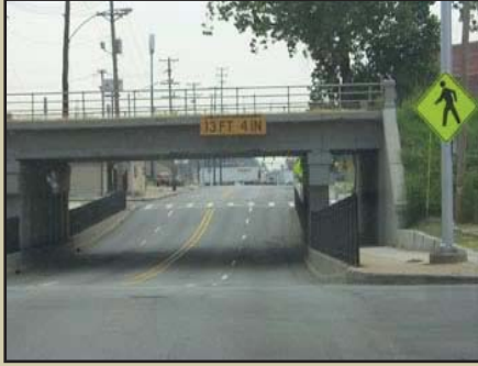
Pedestrian underpass with metal railing for pedestrian safety and separation.
