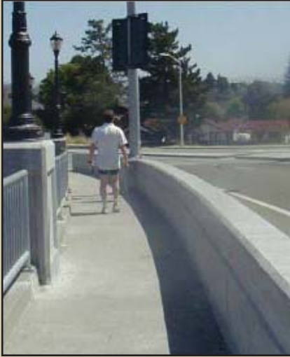
Pedestrian sidewalk on bridge with separation.
