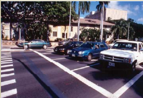
Advance stop bar at a crosswalk; Source: PBIC Image Library
