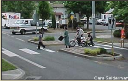
Pedestrian Refuge Island with at-grade crosswalk- credit: www.saferoutes.org
