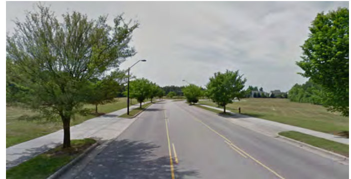
Redford Place Drive is at the upper limit of a typical low-volume collector or residential street. The particular design and infrequent curb cuts of this road might suggest dedicated bicycle lanes; such a prescription would probably preclude a center turn lane due to the costs of relocating utilities, curbing and landscaping that would be necessary were the center turn lane retained. Sharrow markings would be a good intermediate step.
