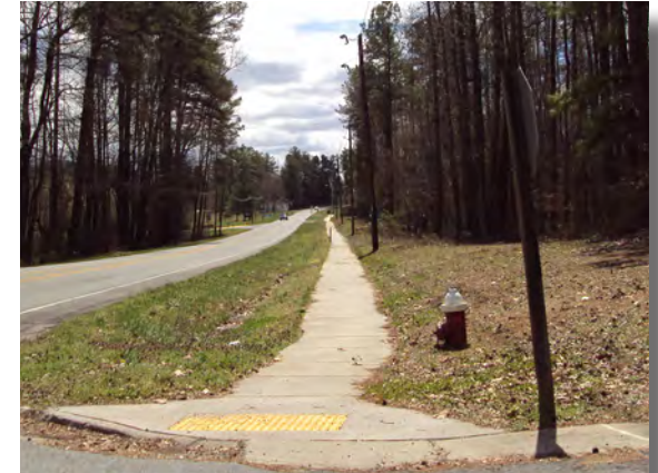
New sidewalk along W. Raleigh Street
