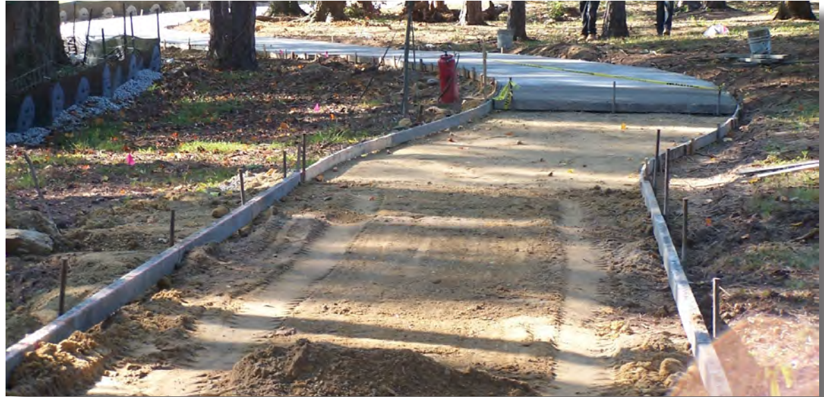
Greenway construction example
