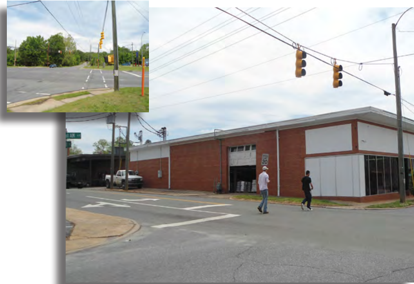
The majority of intersections in Siler City lack crossing treatments, and where crossing treatments do exist, crosswalks are faded and pedestrian signals are not operating properly
