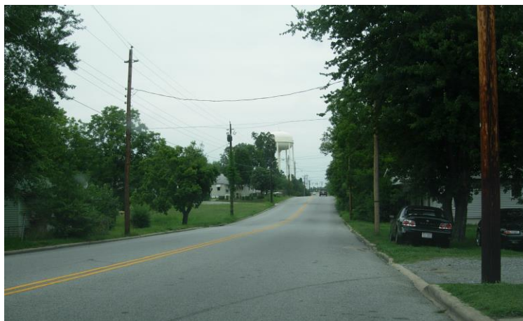
Turner St looking north near intersection with railroad
