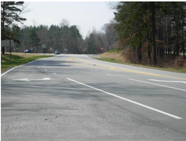
Figure 10 Old Greensboro Road looking southwest towards Business 85
