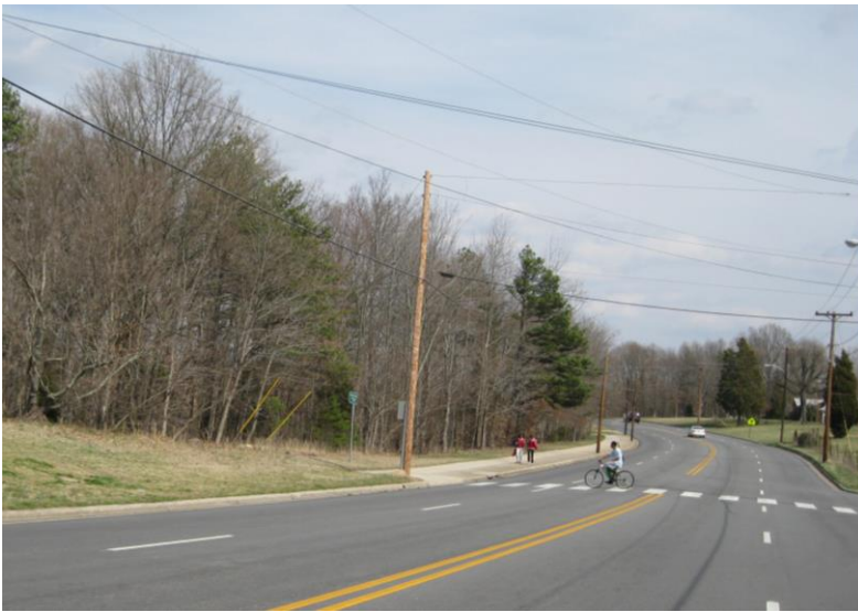
Bicyclist crossing Unity Street where Memorial Park Dr intersects
