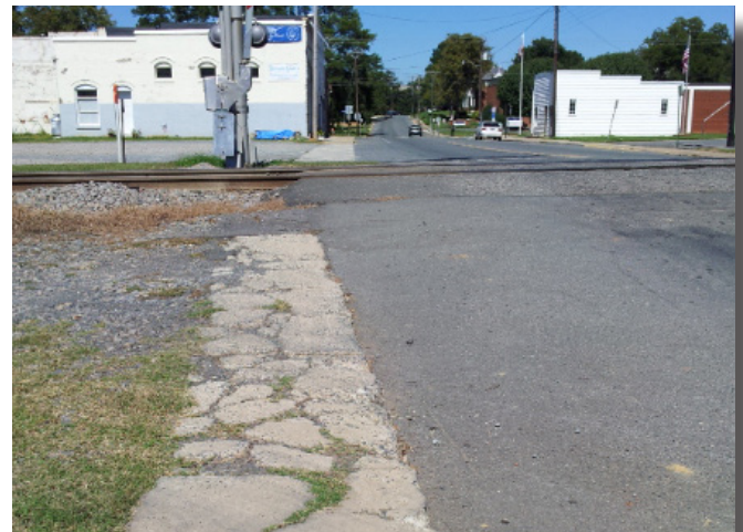
Seaboard RR Tracks & Main St. Intersection: sidewalks and railroad pedestrian crossings are needed
