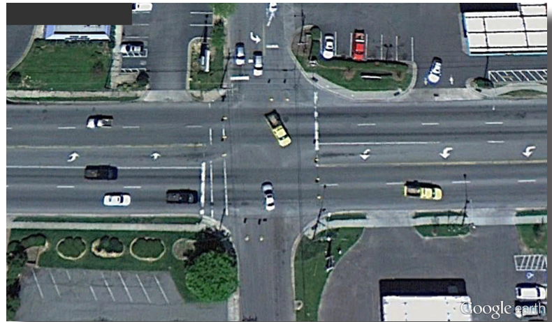
Existing Conditions at Highway 74/Main Street
