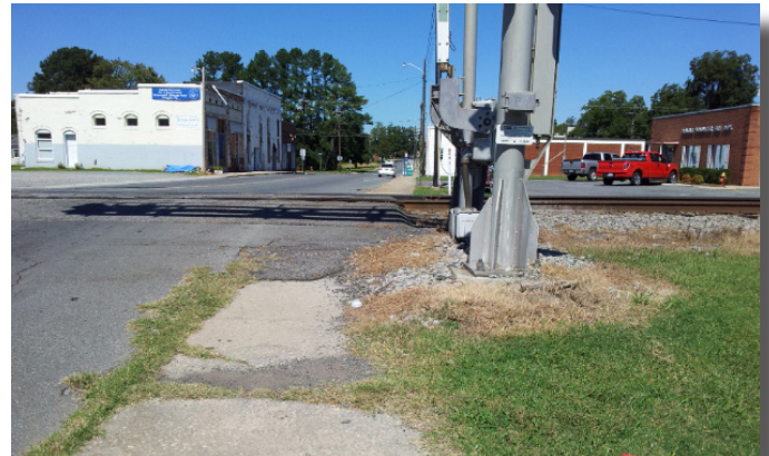
Existing Conditions at Main Street and Seaboard RR Tracks
