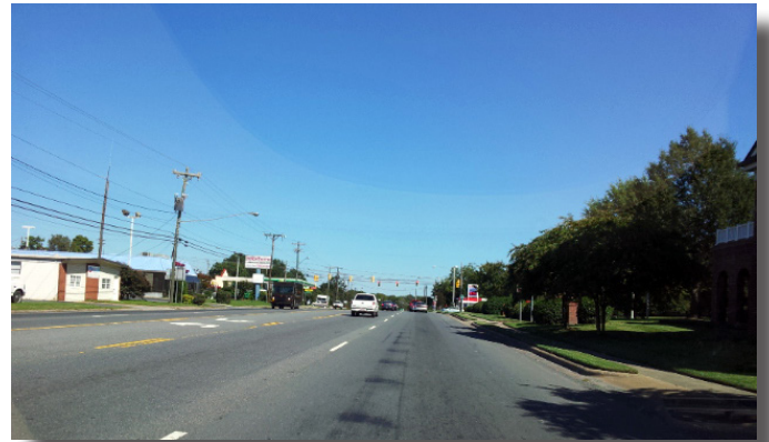
Existing Conditions Along Highway 74
