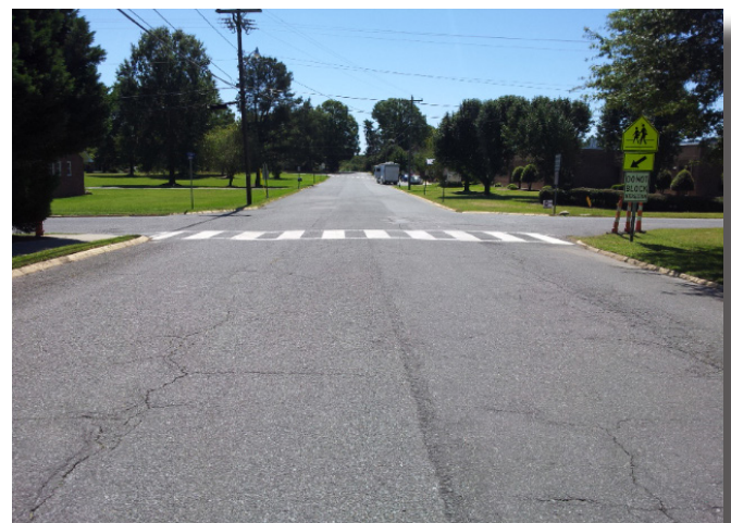
W Elm St. & Bivens St. Intersection: sidewalks along Bivens and Elm Streets and high visibility crosswalks at each intersection leg are needed
