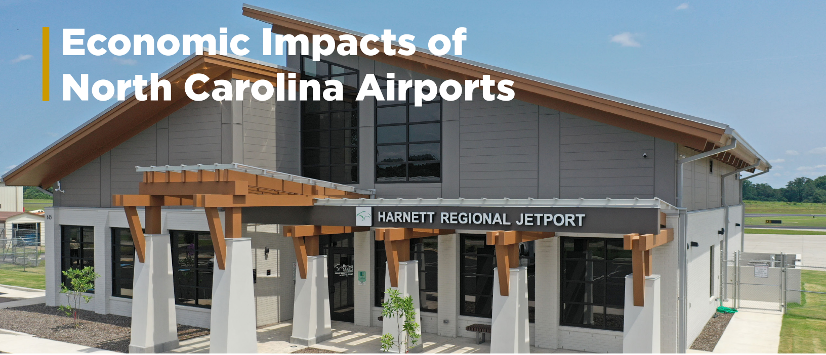
Harnett Regional Jetport unveiled its new 7,000-square-foot state-of-the-art terminal building in June 2024. It provides a modern, comfortable, convenient space for travelers and crew.
