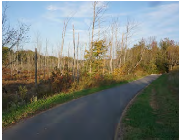
Off Street Greenway/ McAdams
