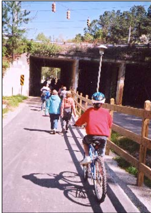
An underpass continues this shared use bicycle path beneath a 4-lane highway with high traffic volume
