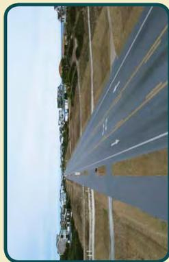
NC 12 3-Lane Widening (90-Foot Right-of-Way) Photo Simulation
