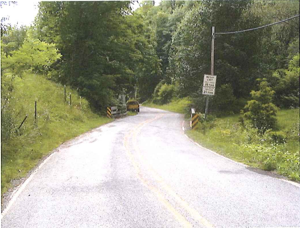
Looking southeast towards bridge.
