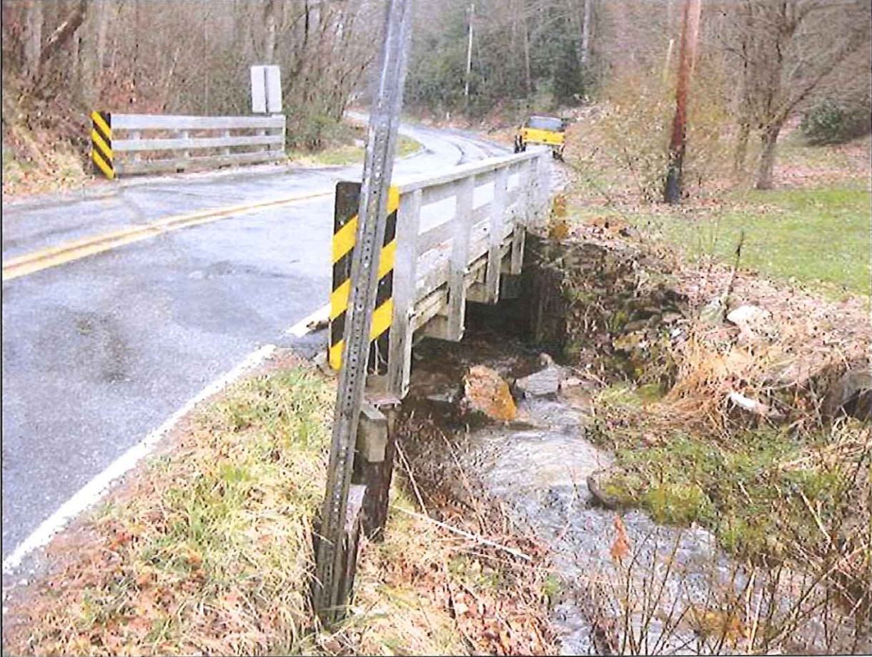
Looking downstream towards bridge.
