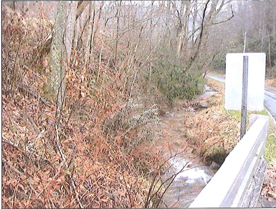
Looking downstream from bridge.
