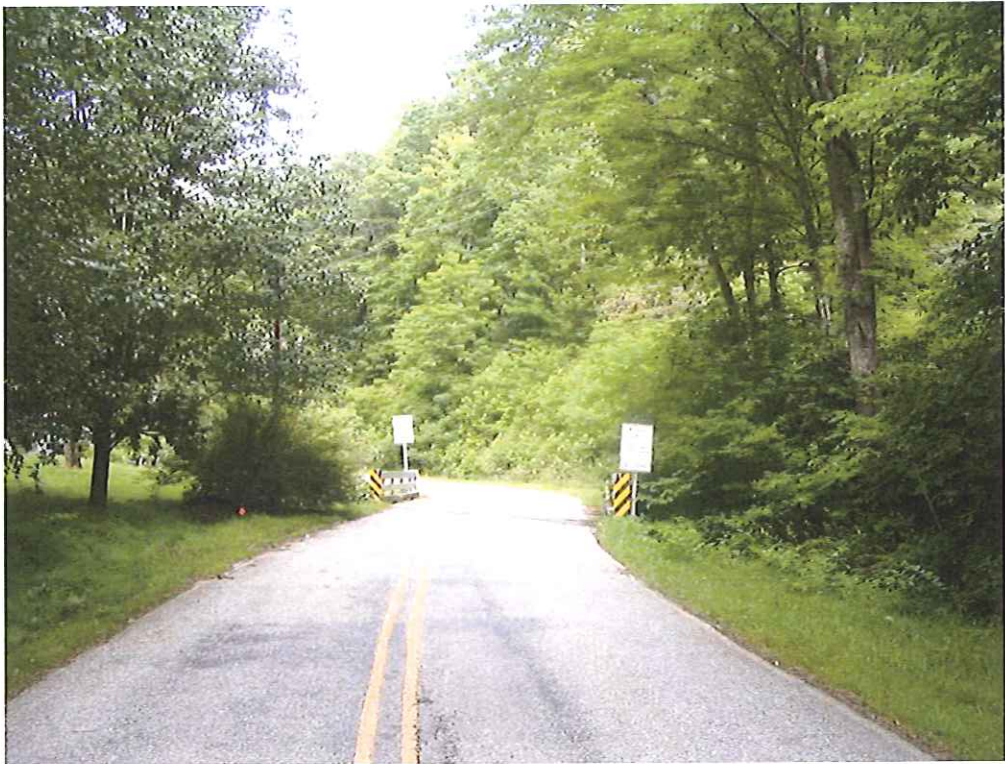
Looking northwest towards bridge.
