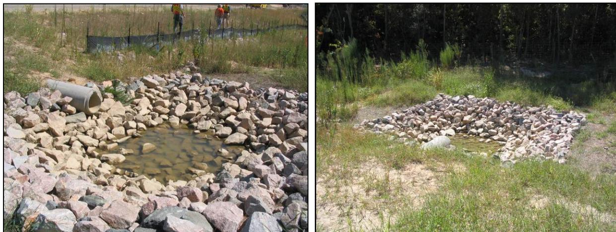
**Figure 4-1.** Preformed scour holes in a linear highway application
