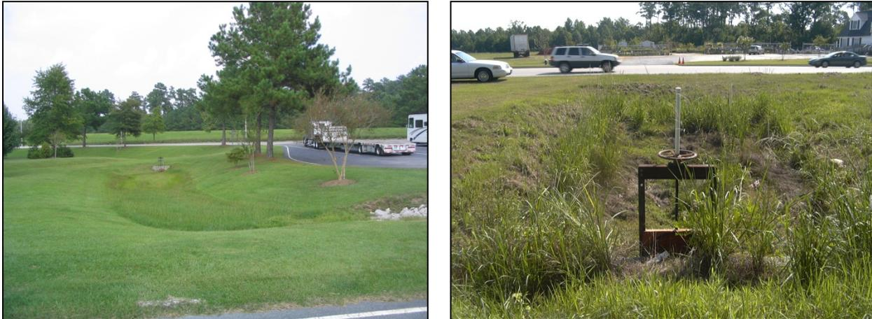
**Figure 8-4.** A hazardous spill basin at a rest area (left) and in a linear highway setting (right)
