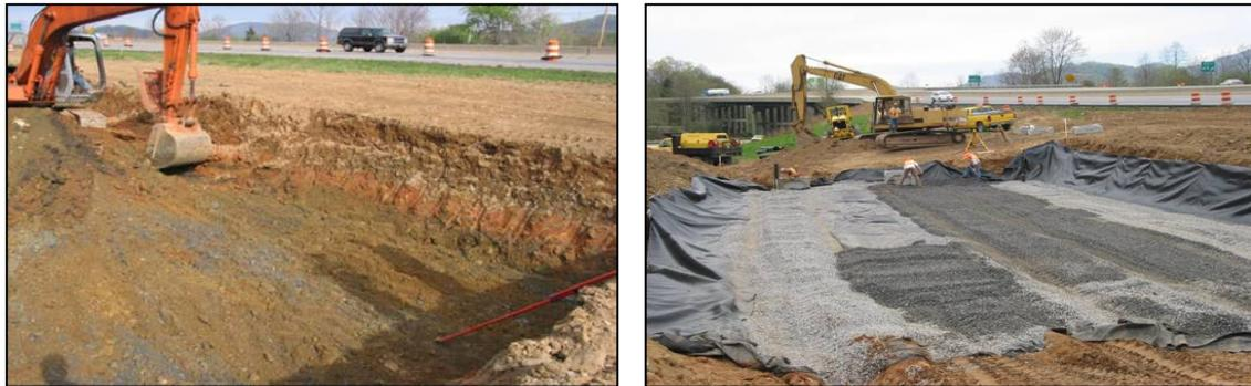
**Figure 2-6.** Bioretention basin during construction
