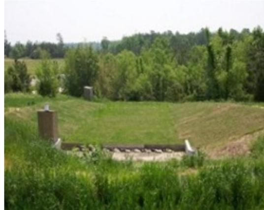
**Figure 2-3.** Bermuda grass filter strip and level spreader
