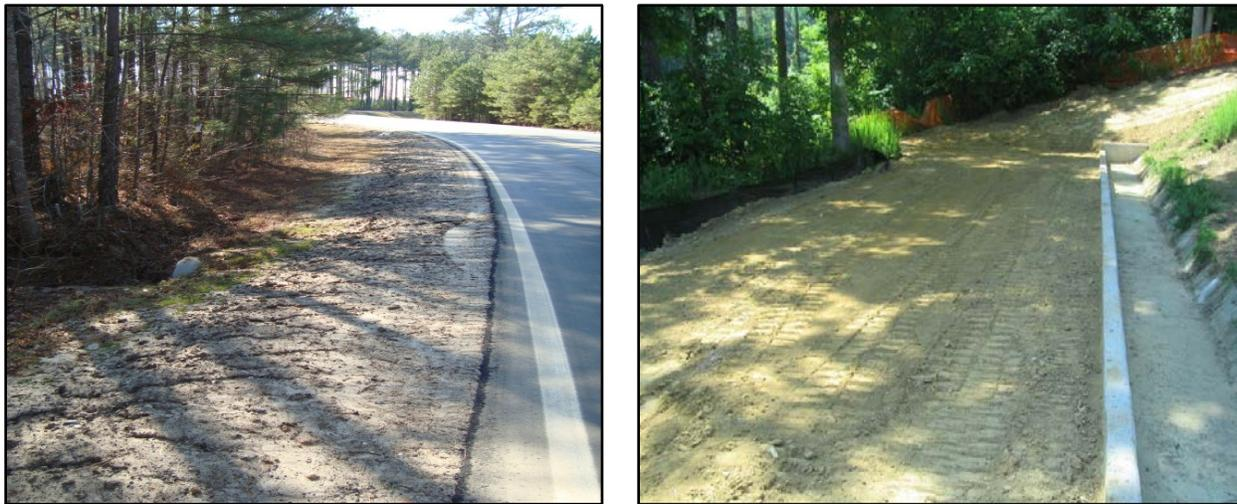
**Figure 14-6.** Filter strips prior to vegetation establishment
