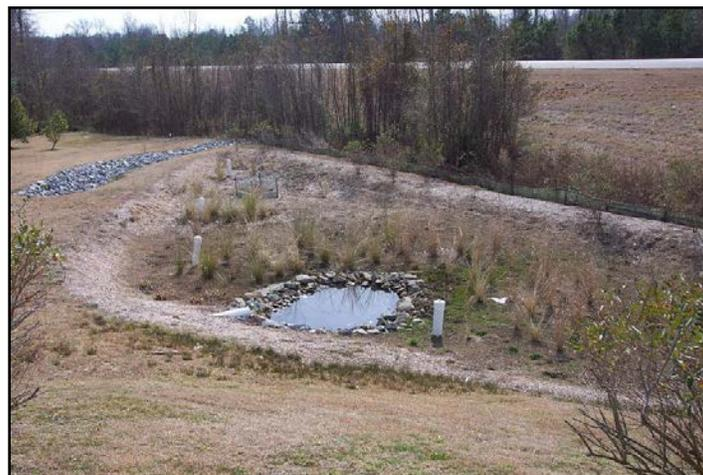
Figure 7-4. Forebay with bioretention basin
