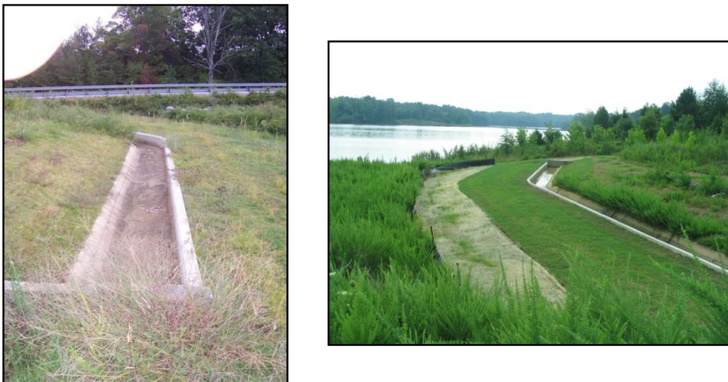
Figure 3-4. Example of a level spreader and buffer system
