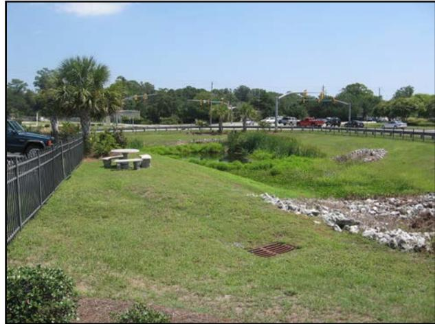
**Figure 12-1.** Typical wet detention basin adjacent to roadway
