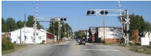
Existing NC 96 (Main Street), Youngsville At Railroad Crossing
