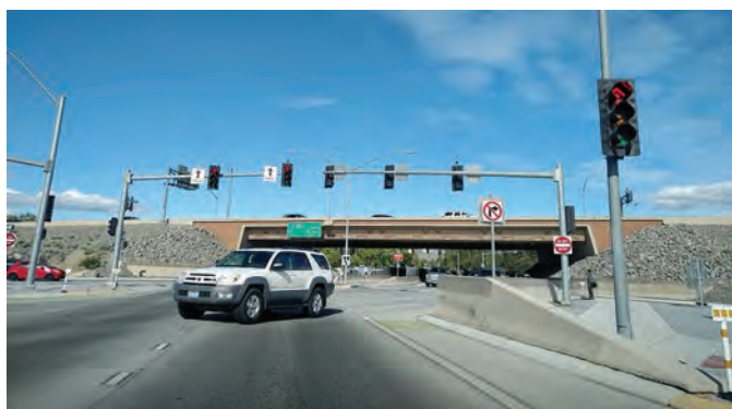
Exhibit 6-68. Barrier application to impede driver sight lines (9).
