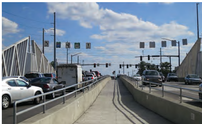
Exhibit 6-38. Example cross section for pedestrian path (Gwinnett County, Georgia) (6).
