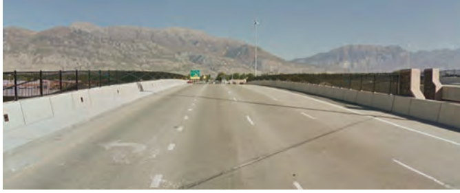
Exhibit 7-10. Use of dotted lines to delineate an exclusive left-turn lane onto a limited access facility (2).
