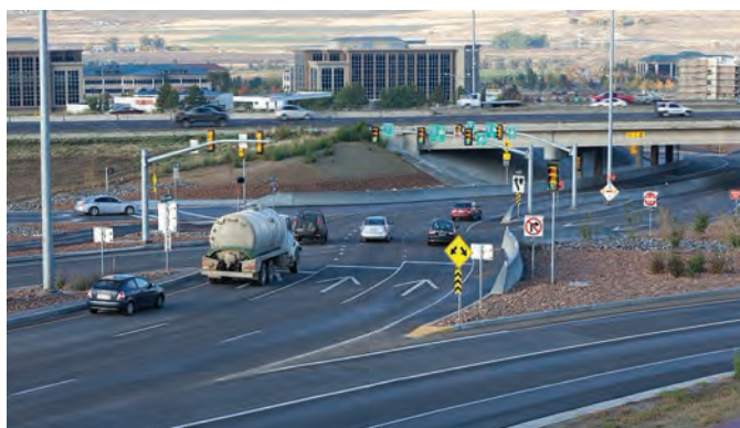
Exhibit 1-6. Crossover location at the DDI located at SR-92 and Interstate 15 (Utah County, Utah) (5).
