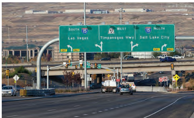
Exhibit 1-7. Overhead signing at the DDI located at SR-92 and Interstate 15 (Utah County, Utah) (5).
