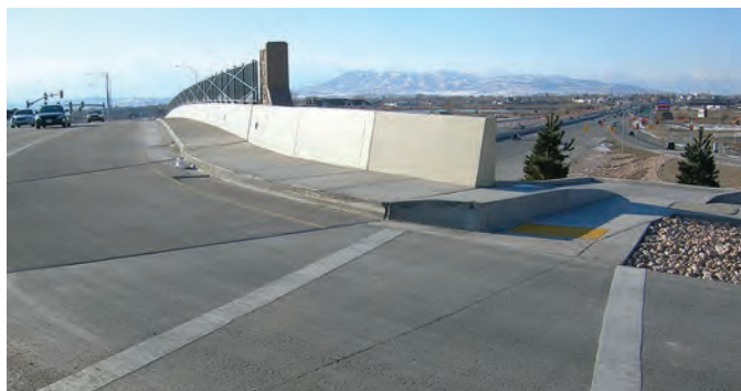
Exhibit 6-51. Pedestrian crossing location at the Pioneer Crossing interchange (American Fork, Utah) (10).
