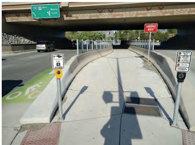
Exhibit 6-53. Median pedestrian crossing and pedestrian treatments at the I-580 and Moana Lane interchange (Reno, Nevada) (9).
