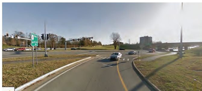
Exhibit 3-18. Outer shared-use path at DDI in Lexington, Kentucky (4).
