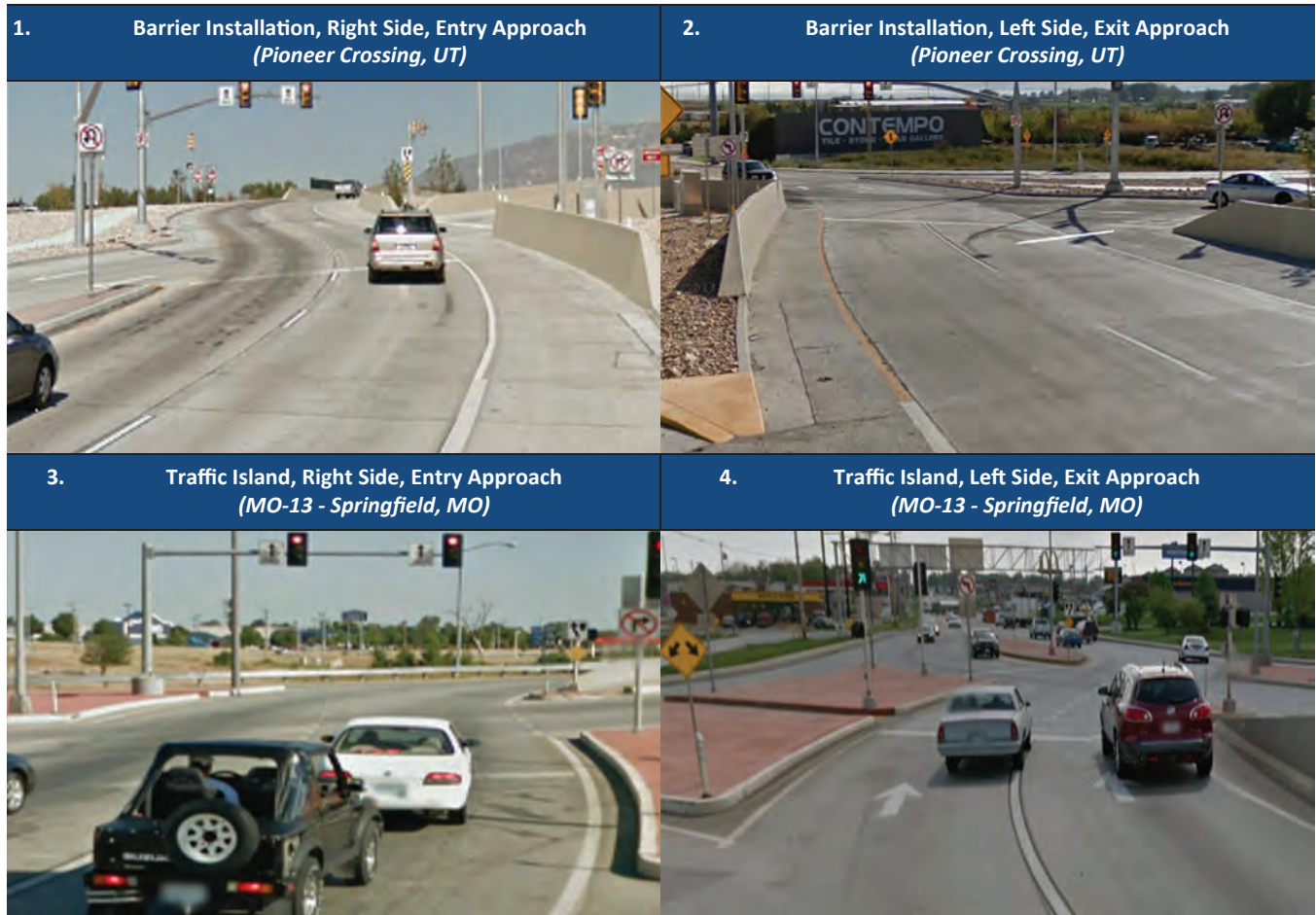
Exhibit 6-69. Examples of barriers and traffic islands to reduce sight lines (3).
