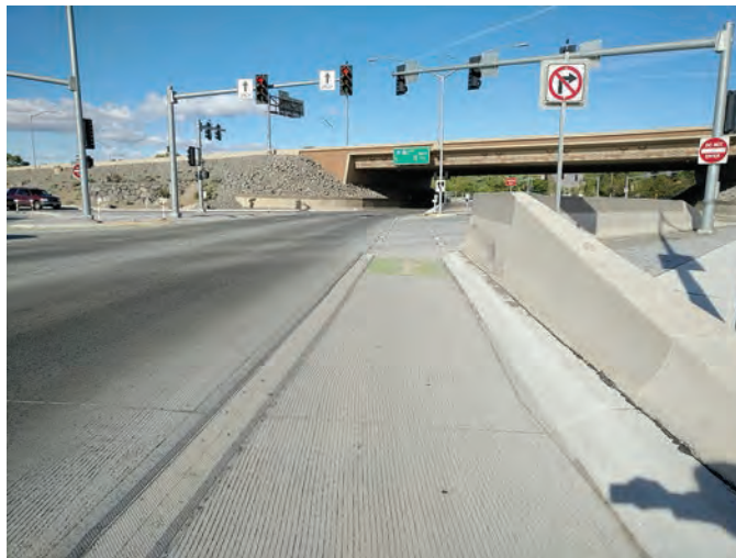
Exhibit 6-33. Tangent crossover intersection at I-580 and Moana Lane (Reno, Nevada) (9).
