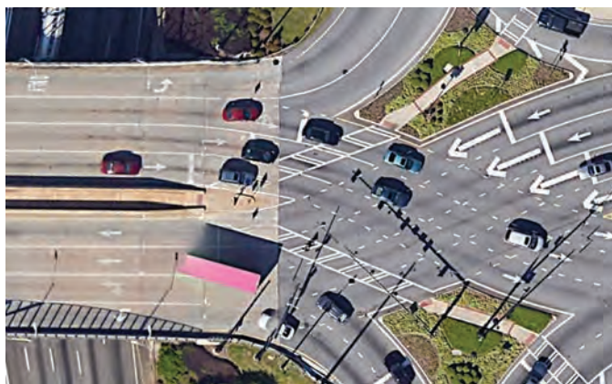
Exhibit 6-25. Example of highly skewed pedestrian crossing (Duluth, Georgia) (5).
