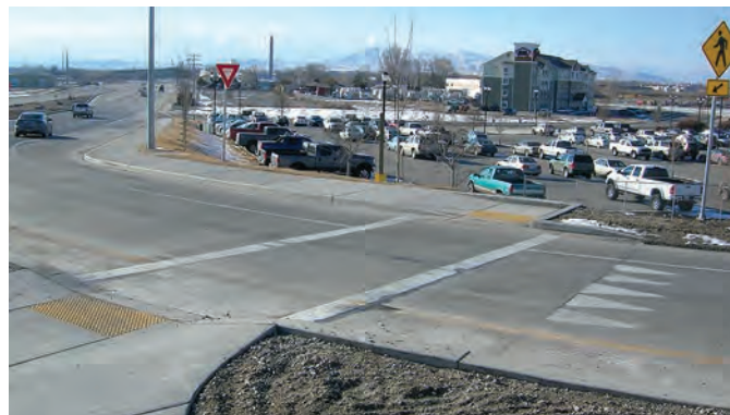
Exhibit 1-8. Pedestrian crossing at the right-turn lane of the exit located at Pioneer Crossing and Interstate 15 DDI (American Fork, Utah) (6).
