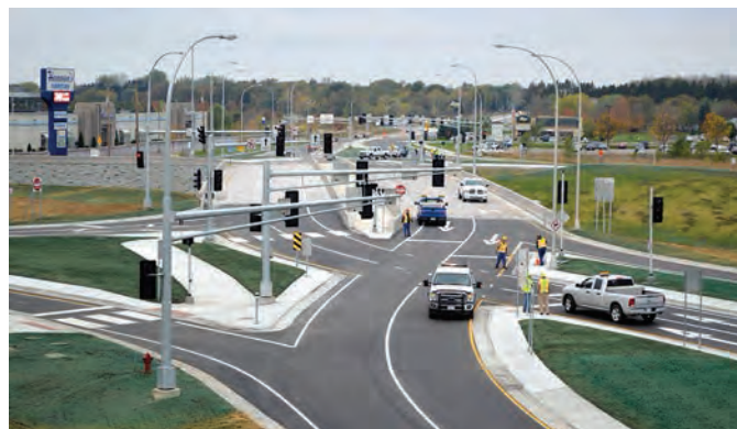
Exhibit 1-4. First constructed DDI in Minnesota at Highway 15 (3).
