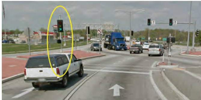
Exhibit 7-22. Supplemental signal on left for an outbound movement at a DDI (2).
