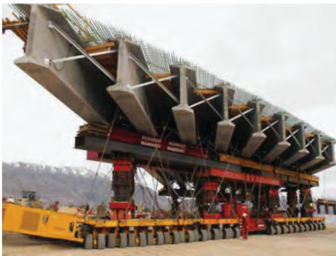
Exhibit 8-1. SPMT brings superstructure to DDI location (3).
