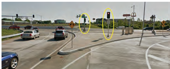
Exhibit 7-23. Supplemental signal for a DDI off-ramp from freeway (2).
