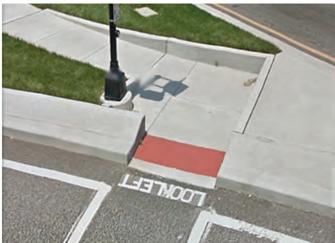
Exhibit 3-54. Engraved pedestrian pavement marking—“Look Left” (4).
