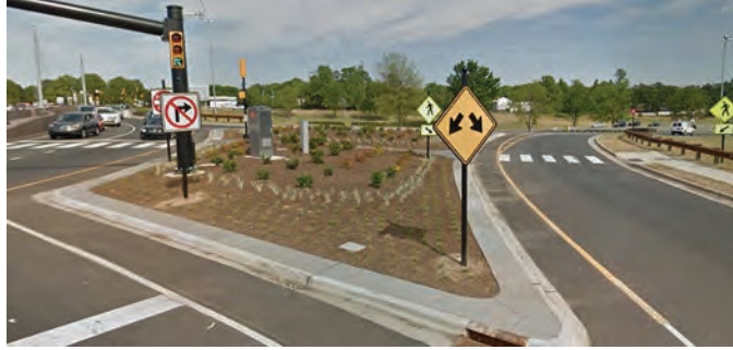
Exhibit 7-15. Signal cabinet located in a landscaped median with good visibility.
