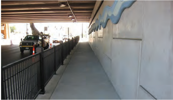
Exhibit 3-2. Outer walkway at Dorsett Road (Maryland Heights, Missouri) (1).
