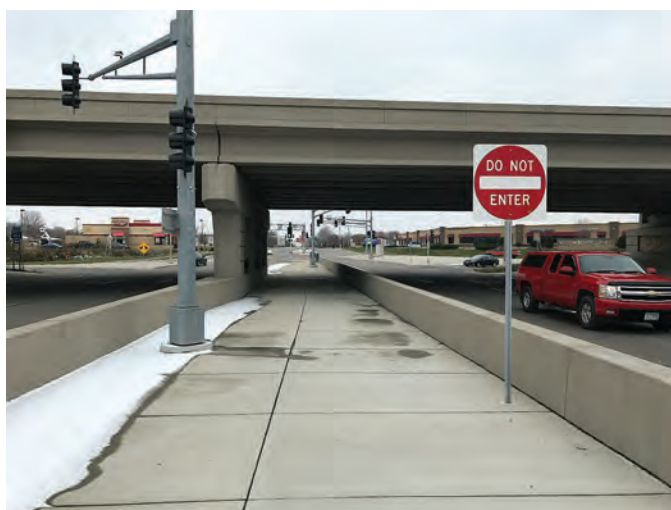
Exhibit 6-39. Pedestrian path at an undercrossing with greater width at the MN-101 and 140th Street interchange (Rogers, Minnesota) (6).
