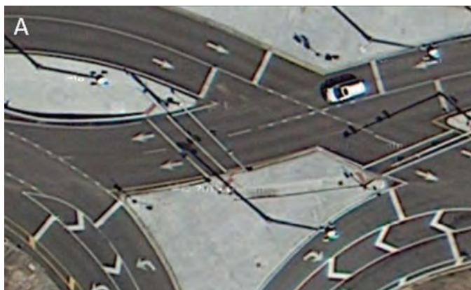
Exhibit 7-13. Staggered stop bar locations at the intersection crossover and exit ramp terminal (2).
