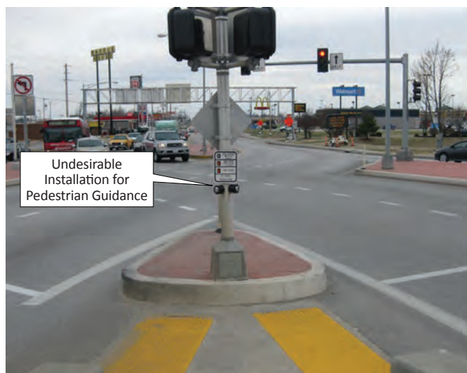
Exhibit 7-25. Undesirable use of single pole with two pedestrian push buttons, no APS, and insufficient separation of the two detectable warning surfaces (2).
