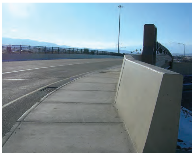
Exhibit 6-52. Pedestrian crossing sight line at the Pioneer Crossing interchange (American Fork, Utah) (10).
