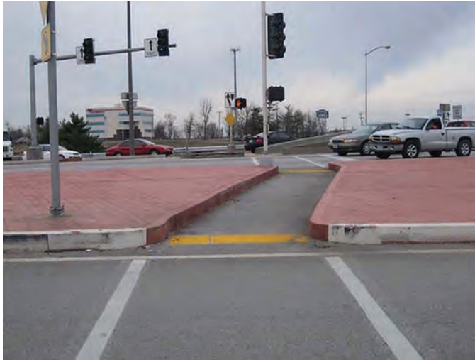
Exhibit 3-49. Example of pedestrian wayfinding provision at DDI via curbing (4).
