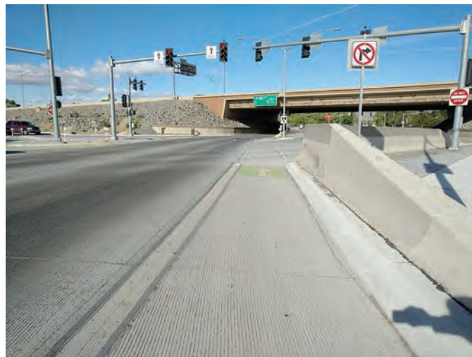
Exhibit 6-48. Bicycle lane approaching the DDI crossover at I-580 and Moana Lane (Reno, Nevada) (9).
