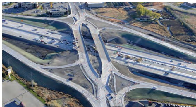
Exhibit 1-10. DDI (overpass) at 500 East American Fork (American Fork, Utah) (1).
