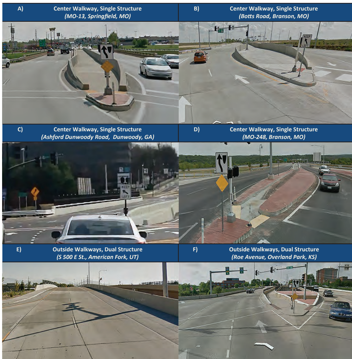
Exhibit 6-45. Examples of various overpass cross sections (3).
