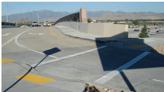
Exhibit 3-53. Example of pedestrian crossing at free-flow left onto freeway (8).
