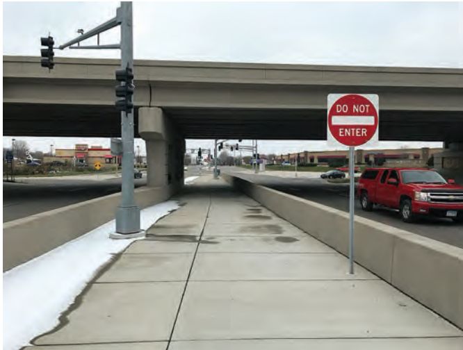
Exhibit 6-46. Undercrossing at the MN-101 and 140th Street interchange (Minnesota) (6).
