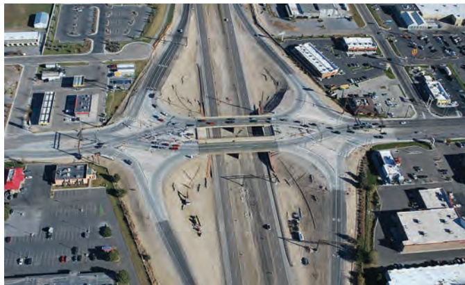
Exhibit 1-5. First constructed DDI in Idaho at Interstate 86 and US-91/Yellowstone Highway (Pocatello-Chubbuck, Idaho) (4).
