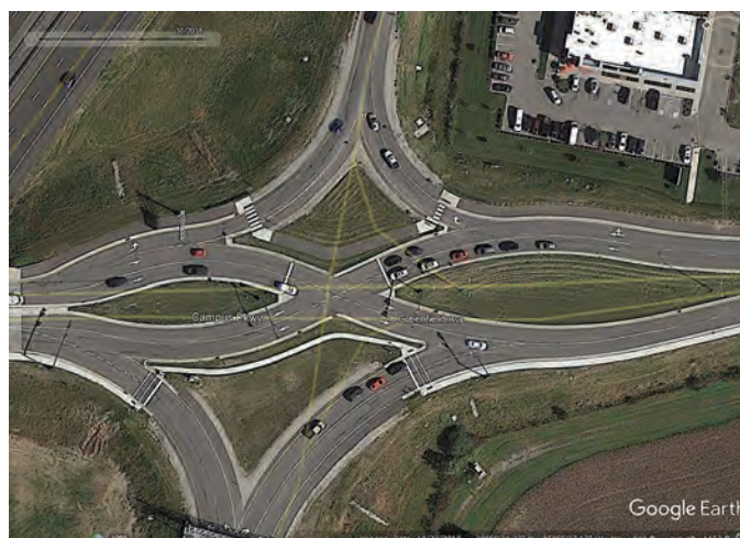
Exhibit 6-42. Tangent crossover configuration at I-69 and Campus Parkway interchange (Fishers, Indiana) (5).
