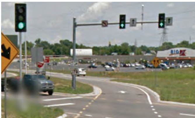
Exhibit 7-17. Type 2 crossover signals with a Type 1 supplemental signal on left (2).
