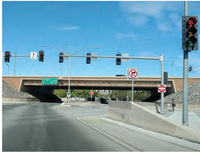
Exhibit 3-16. Bicycle lane extending through inbound crossover (3).
