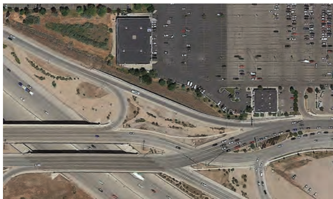
Exhibit 6-22. Effects of skew at Pioneer Crossing interchange (American Fork, Utah) (5).
