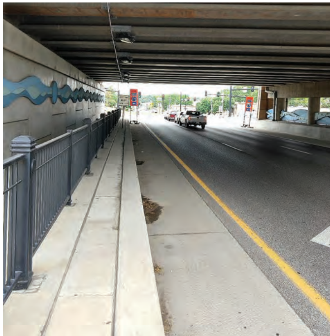
Exhibit 6-10. Example vertical wall and sidewalk (Maryland Heights, Missouri) (2).
