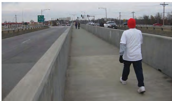
Exhibit 3-1. Inner walkway at MO-13 (Springfield, Missouri) (1).
