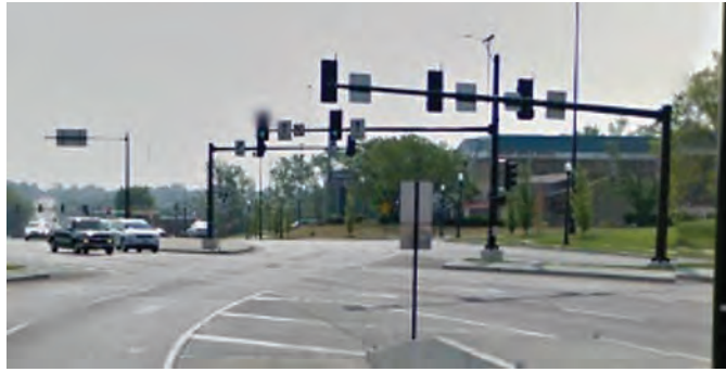
Exhibit 7-20. Mast arm assembly limiting approach visibility (2).
