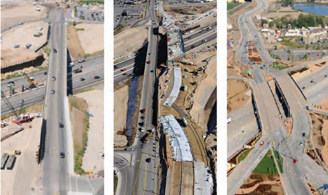
Exhibit 8-2. Construction staging using pre-cast construction methods (5).
