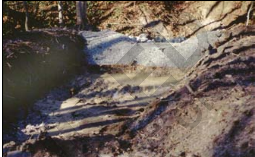
Figure 28. Rock Silt Check Type “A”
