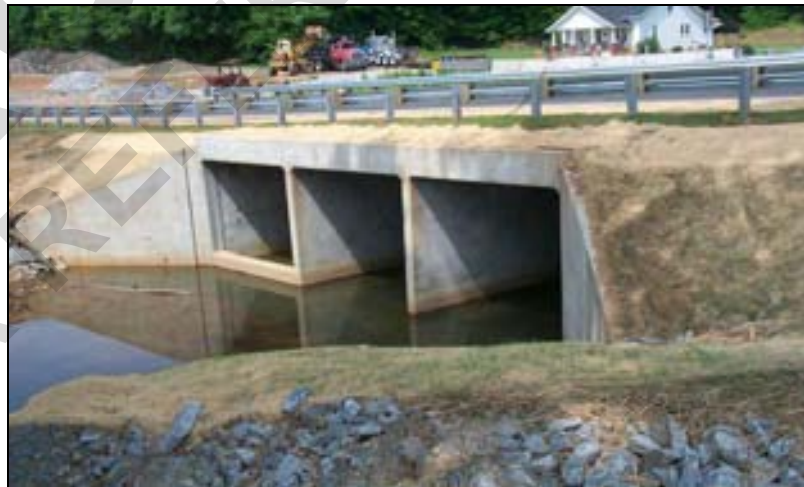
Figure 9. Completed Culvert Extension
