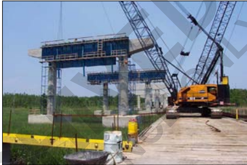
Figure 21 – Bridge Construction within Wetlands
