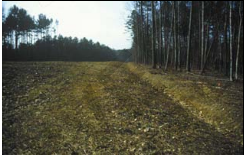
Figure 27. Temporary Silt Ditch
