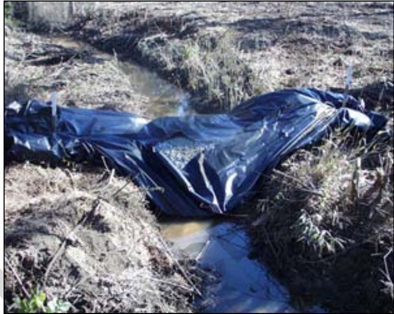
Figure 34. Installation of Stone with Impervious Fabric
