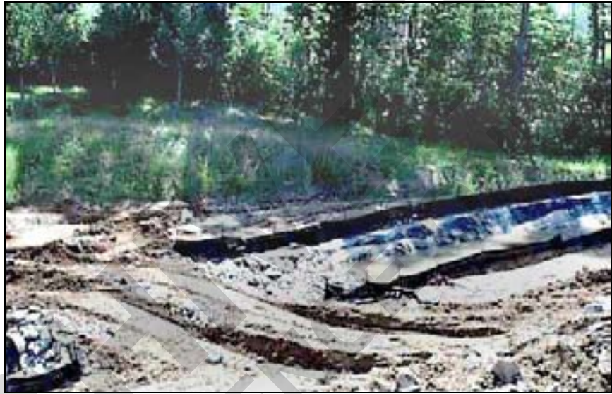
Figure 41. Temporary Piped Crossing
