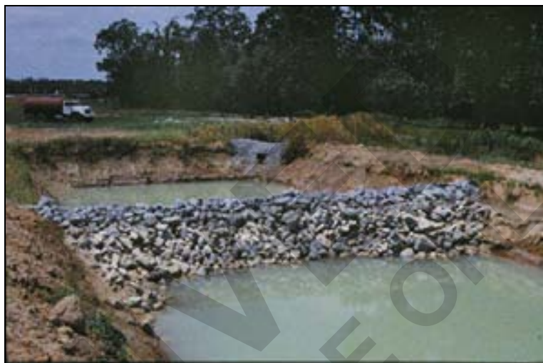
Figure 38. Stilling Basin for Pumped Effluent
