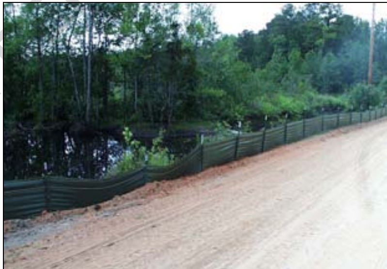
Figure 1. Typical Perimeter Erosion Controls
