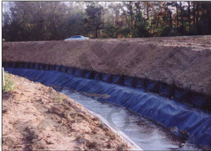
Figure 32. Fabric Lined Diversion Channel
