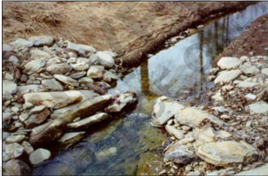
Figure 49. Cross Vane Rock Weir (looking upstream)
