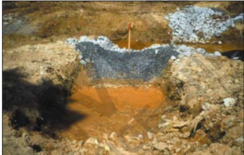
Figure 29. Temporary Rock Sediment Dam Type “B”
