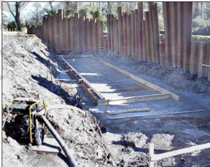
Figure 11. Pipe/Culvert Foundation Installation
