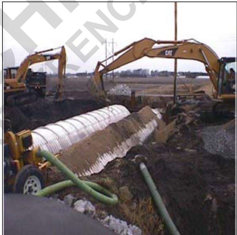
Figure 12. Pipe/Culvert Installation
