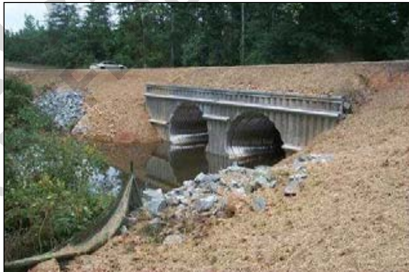
Figure 18. Completed Headwall Installation
