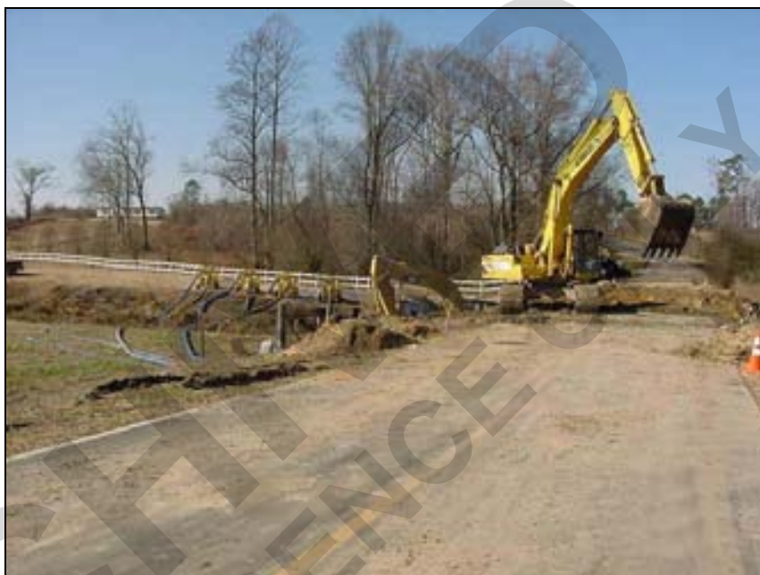
Figure 30. Bypass Pumping
