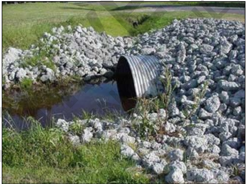
Figure 13. Pipe/Culvert Outlet Protection
