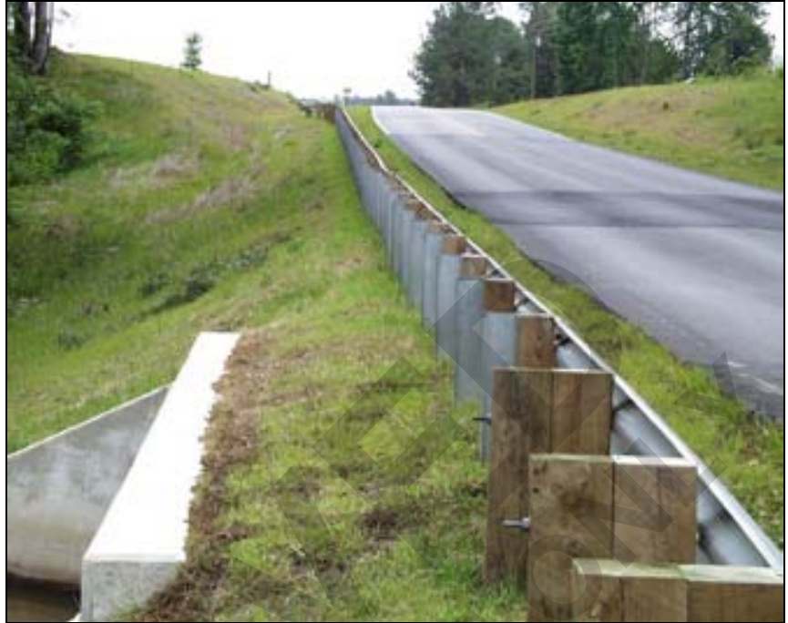
Figure 14. Completed Pipe/Culvert Installation
