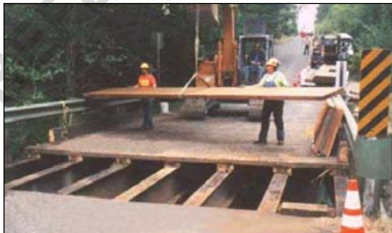
Figure 20. Bridge Demolition
