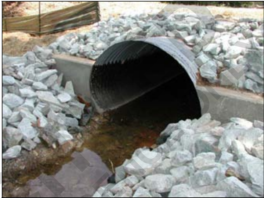
Figure 47. Riprap Outlet Protection
