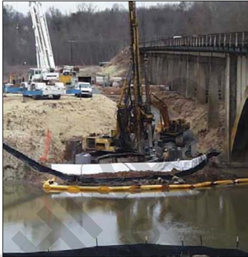
Figure 4 – Managing the Work Area
