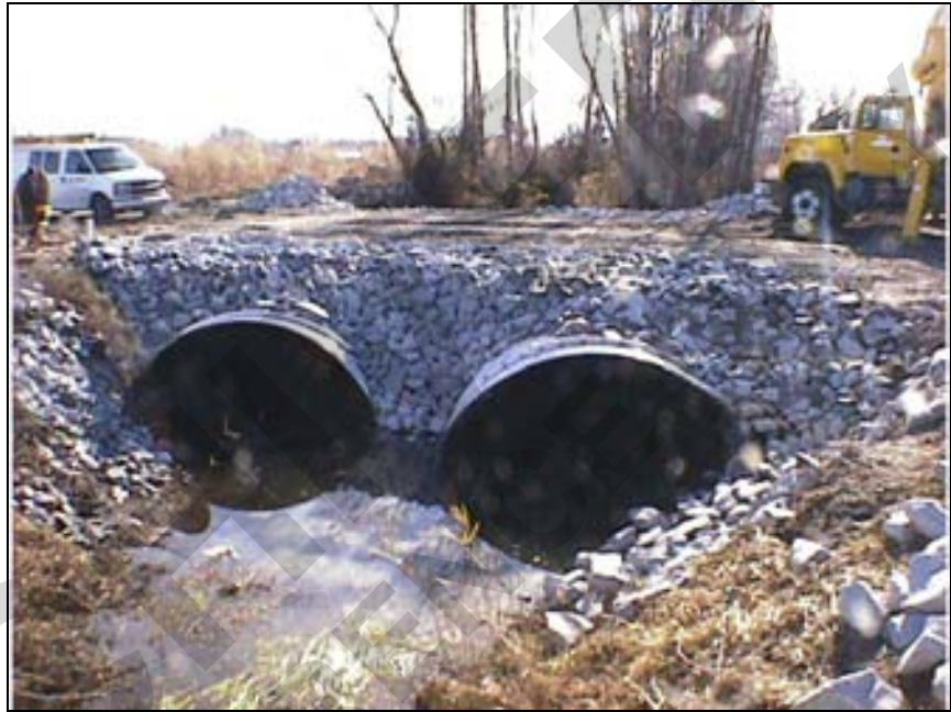
Figure 46. Riprap Slope Protection
