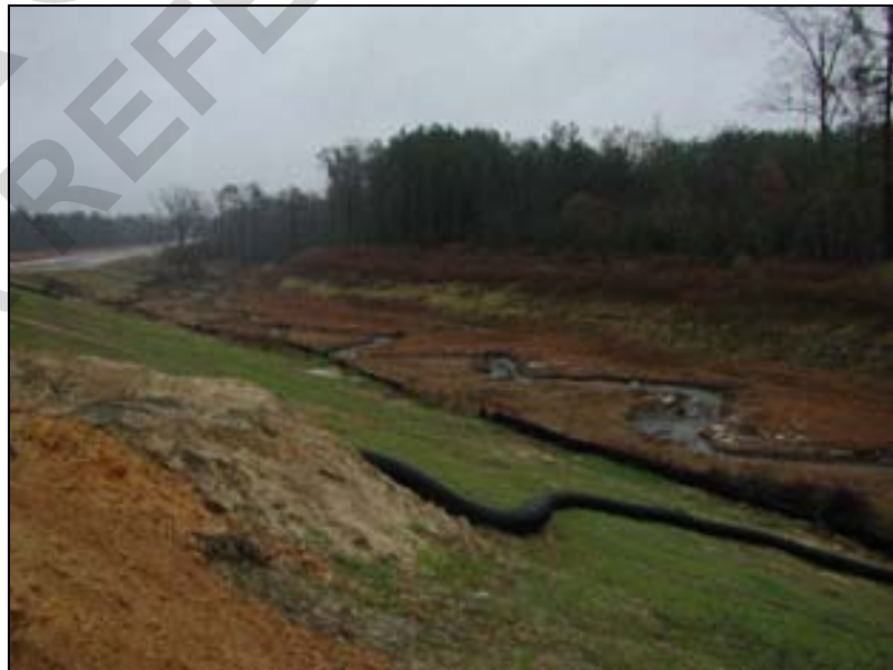
Figure 24. Completed Stream Channel Relocation
