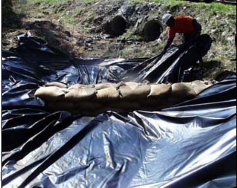
Figure 35. Sand Bag Installation
