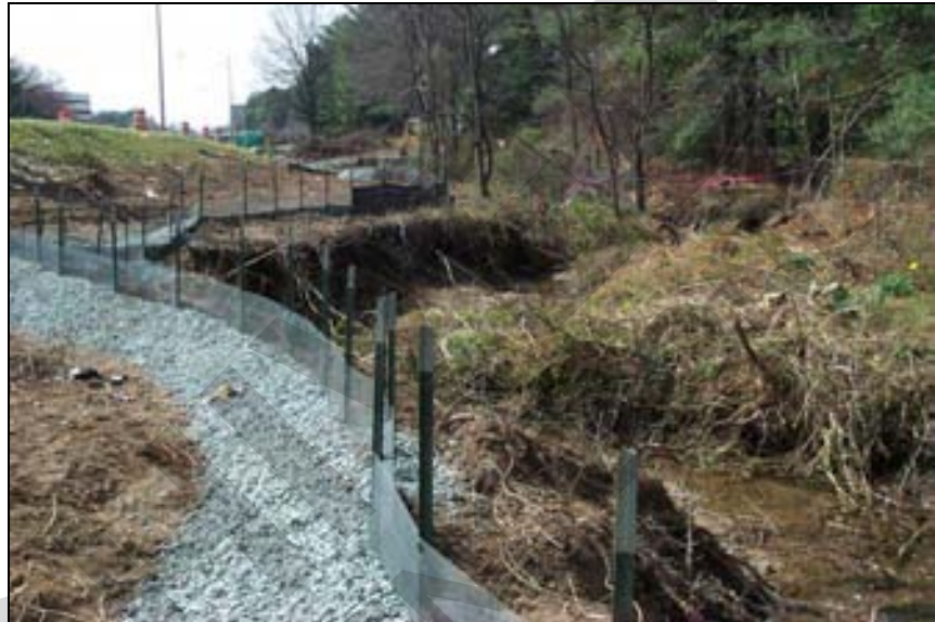
Figure 26 – Typical Special Sediment Control Fence
