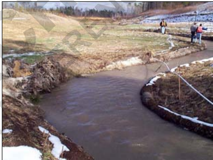
Figure 23. Stream Channel Relocation
