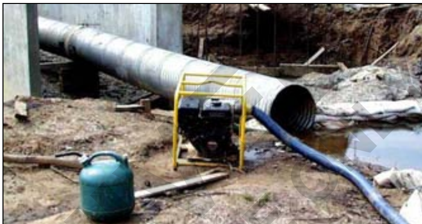
Figure 31 Suspended Bypass Pipe
