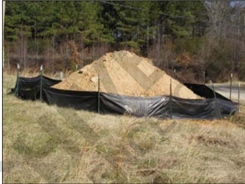
Figure 5. Typical Spoil Management
