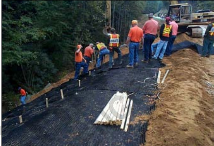
Figure 45. Erosion Control Blankets
