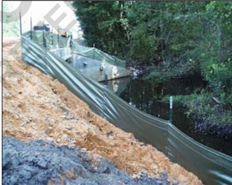
Figure 16. Headwall BMP Installation
