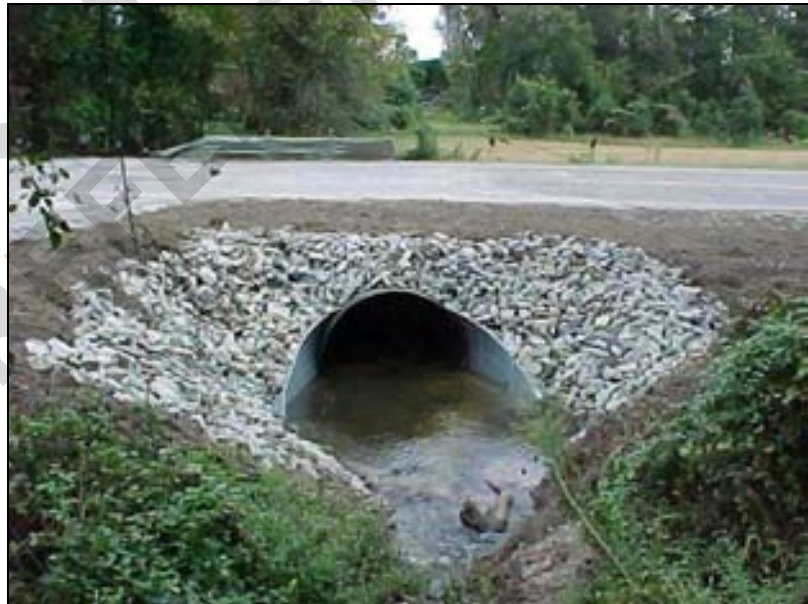
Figure 19. Completed Outlet Maintenance
