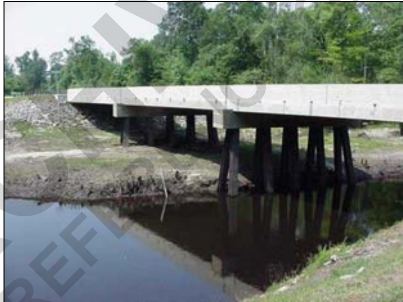
Figure 22. Completed Bridge Construction
