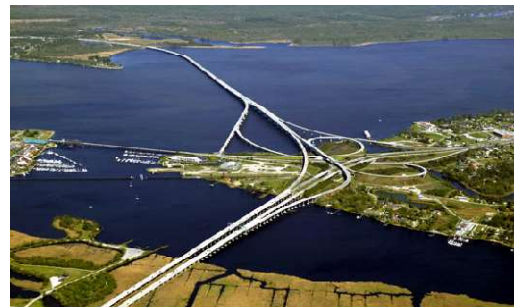
Neuse River Bridge, New Bern - NC
