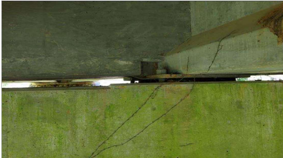
(DRONE PHOTO) TYPICAL BEARING UNDER BEAM 3 AT INTERIOR BENT 2
