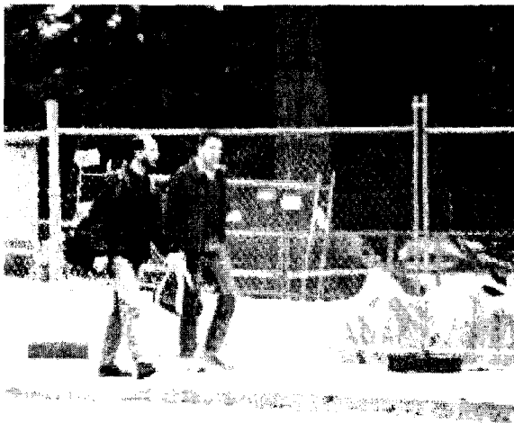
Fencing used to secure a work area supported by blocks needs to be positioned to avoid creating obstacles or tripping hazards for pedestrians.
