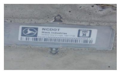
Replaces the NCDOT stamping process with a 3 in 1 tag. Tag can be read visually, via an RFID scanner, or a Barcode reader.
