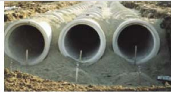
Good amount of loose compressible material
