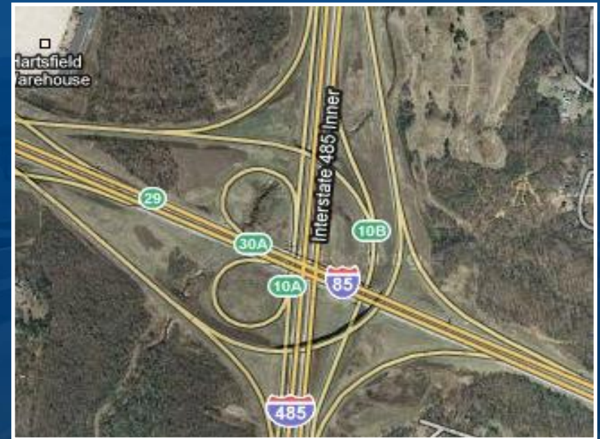
Modified Clover Interchange I-85 and I-485 (18 miles south of R2123-CE site), built by Lane/Rea for NCDOT
