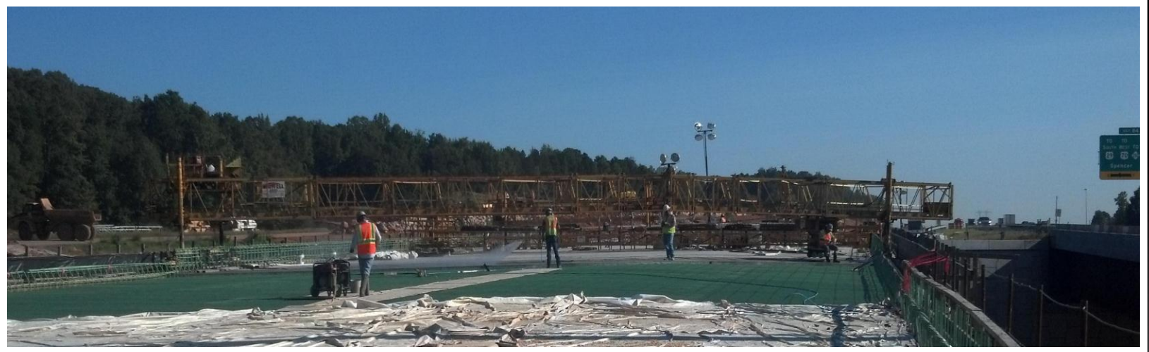
Bridge Deck Construction
