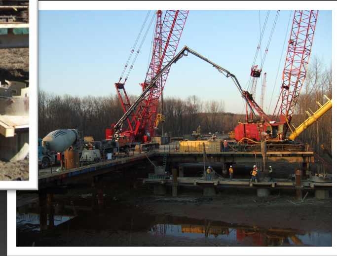
Foundation Installation
