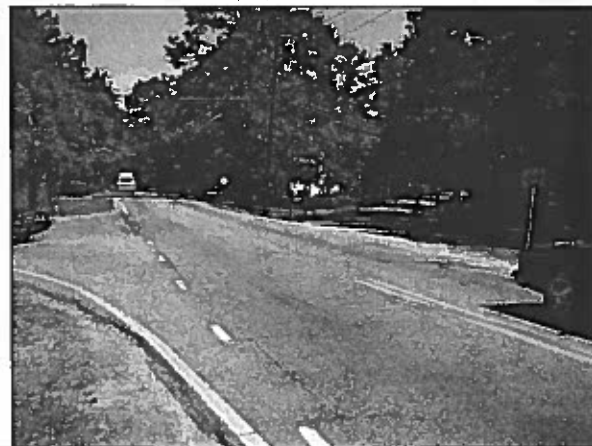
Photo 5 - NC 5 Northbound at Linden Road
