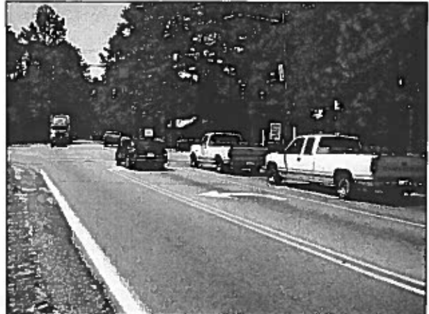
Photo 8 – NC 5 Southbound at Morganton Road
