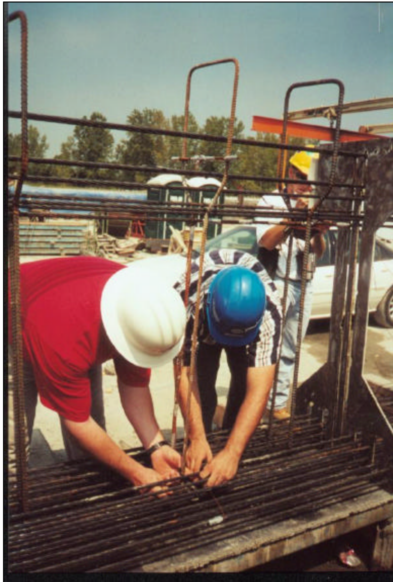
Figure 3.26 Installing Thermocouples
