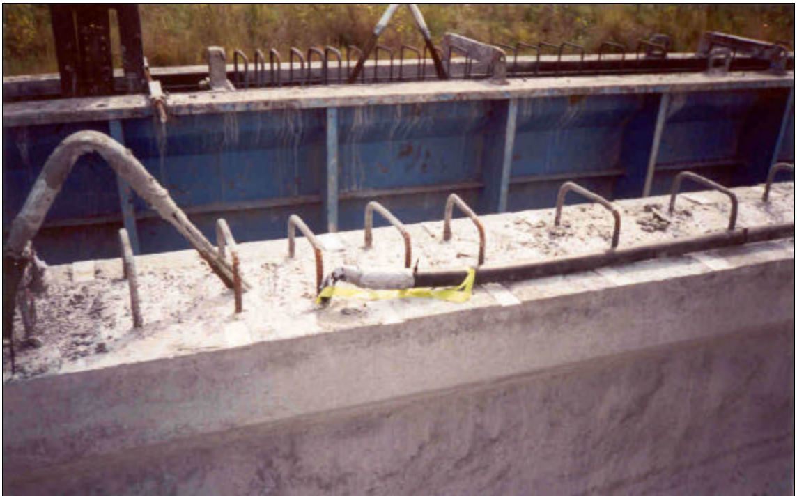
Figure 3.36 Protection of Lead Wires Exiting Girder
