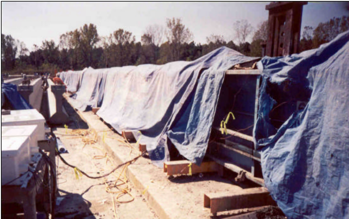
Figure 3.35 Covered Casting Bed
