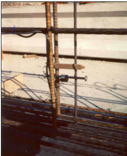
Figure 3.30 Embedment ERSG and VWG at Mid-span
