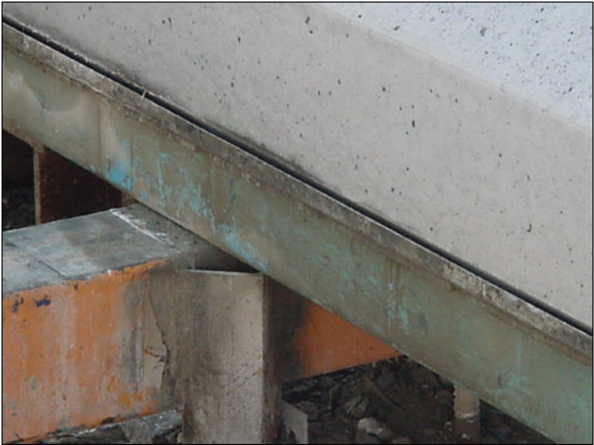
Figure 3.96 Camber of Girder D4
