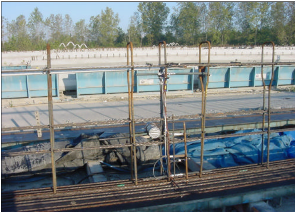
Figure 3.32 All Gages in Place at Mid-span
