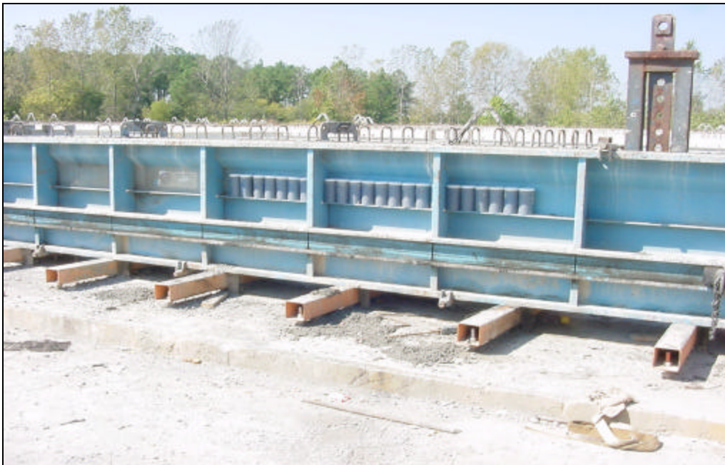
Figure 2.2 Specimen Curing Before Placement of Tarp and Moist Cure
