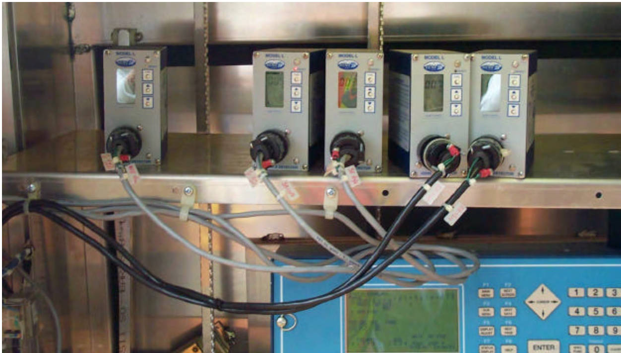
Shelf-mounted detector amplifiers with secondary count outputs
