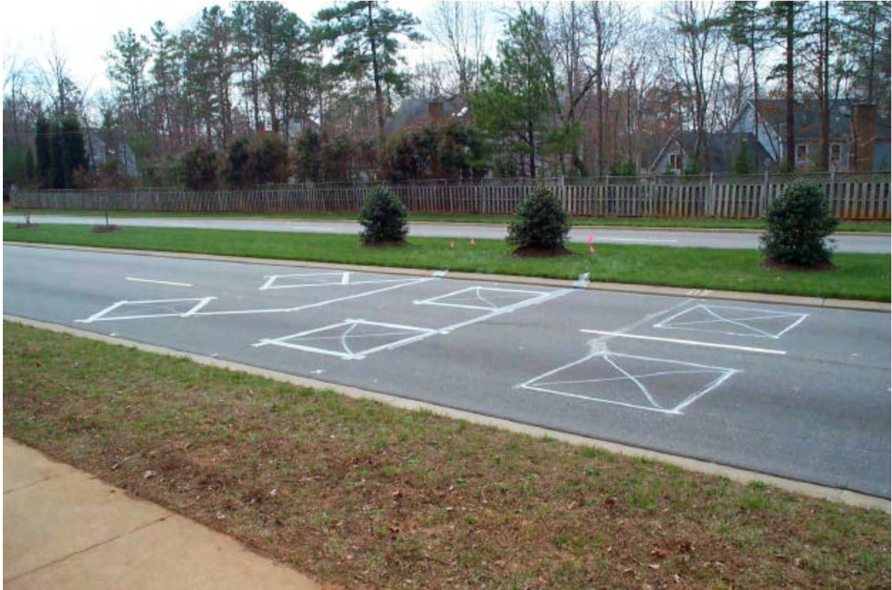
Westbound Cary Parkway: temporary diamond, temporary square, and permanent square signal detector loops
