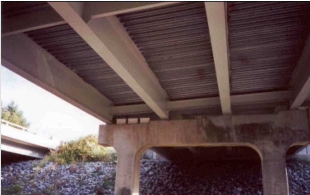
Figure 4.12 Instrumentation boxes at project site.
