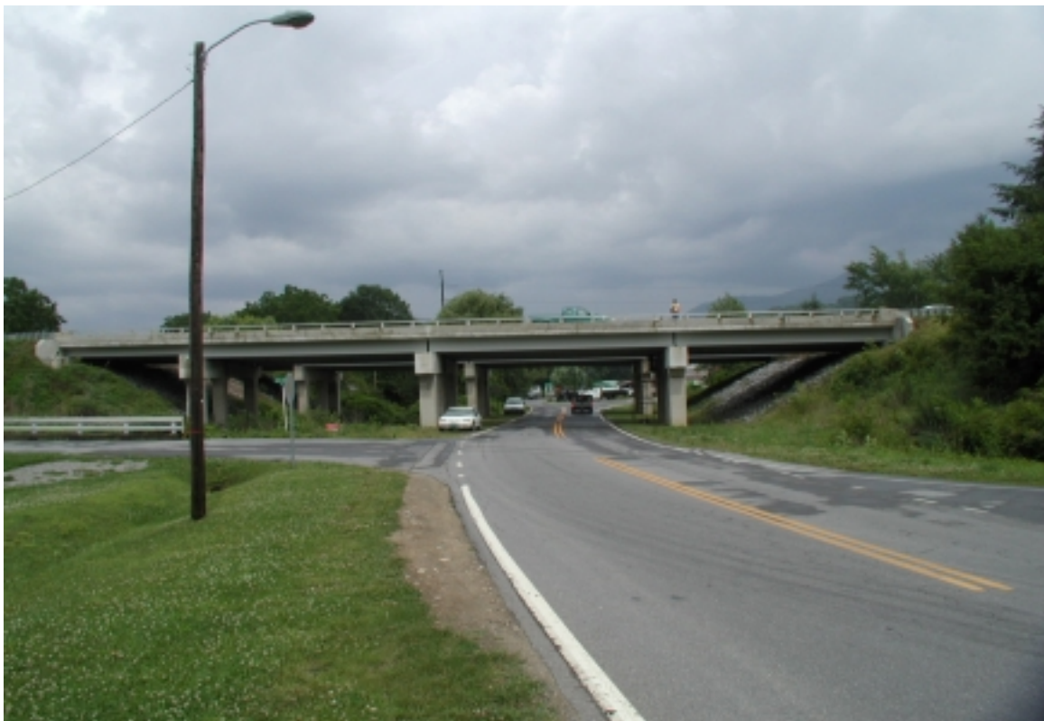
Figure 1.2 Bridge elevation, looking east.
