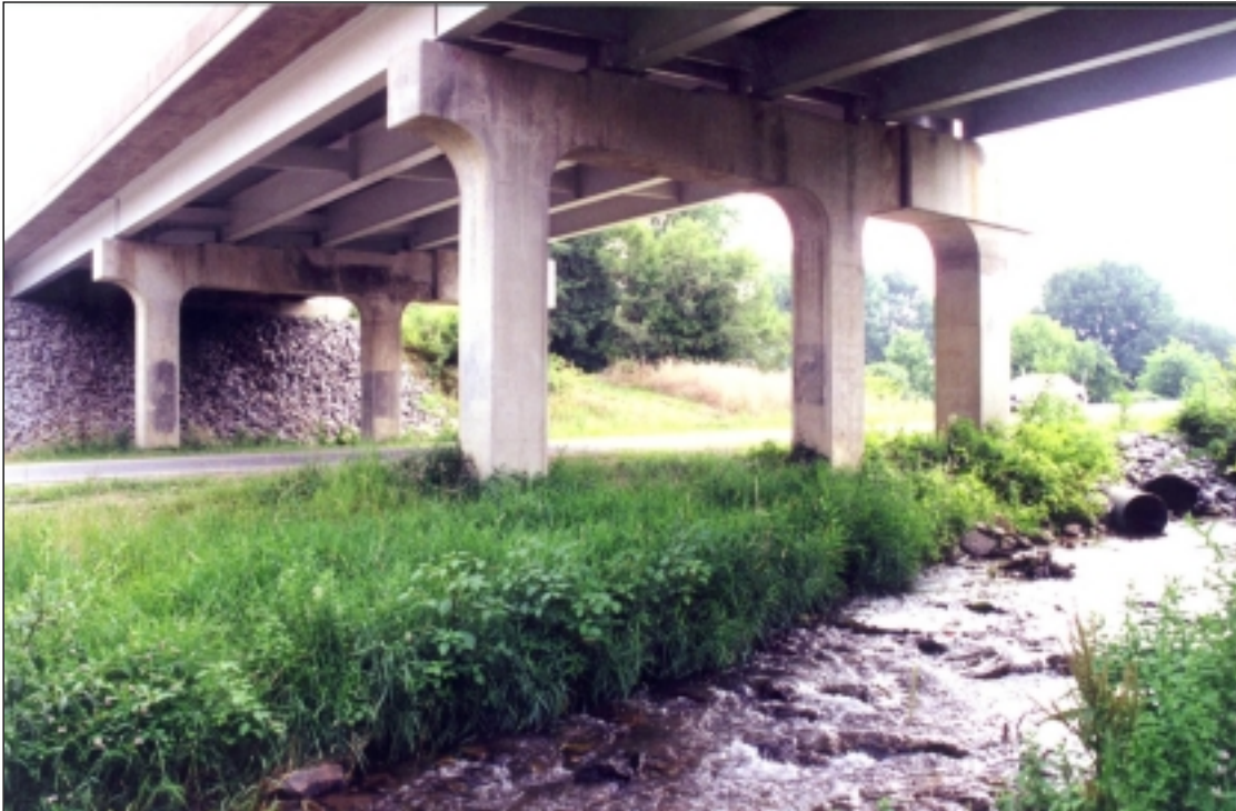
Figure 1.3 Plott Creek and underside of bridge.
