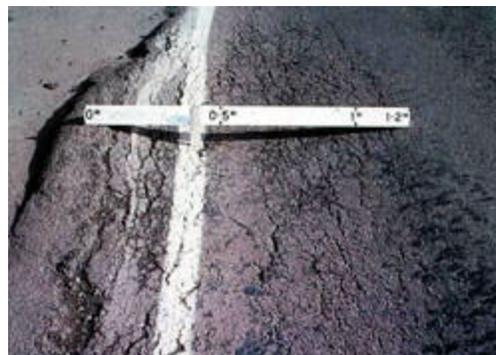
**Figure 1-3 Distortion and shoving, deformation of surface layer under load**
