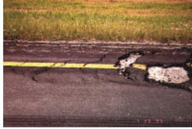
**Figure 1-1 Delamination of surface course**
