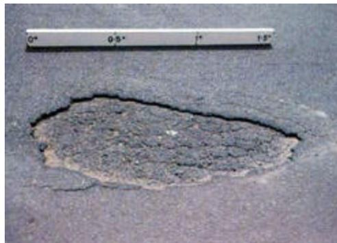
**Figure 1-2 Delamination, exposure of underlying layer**
