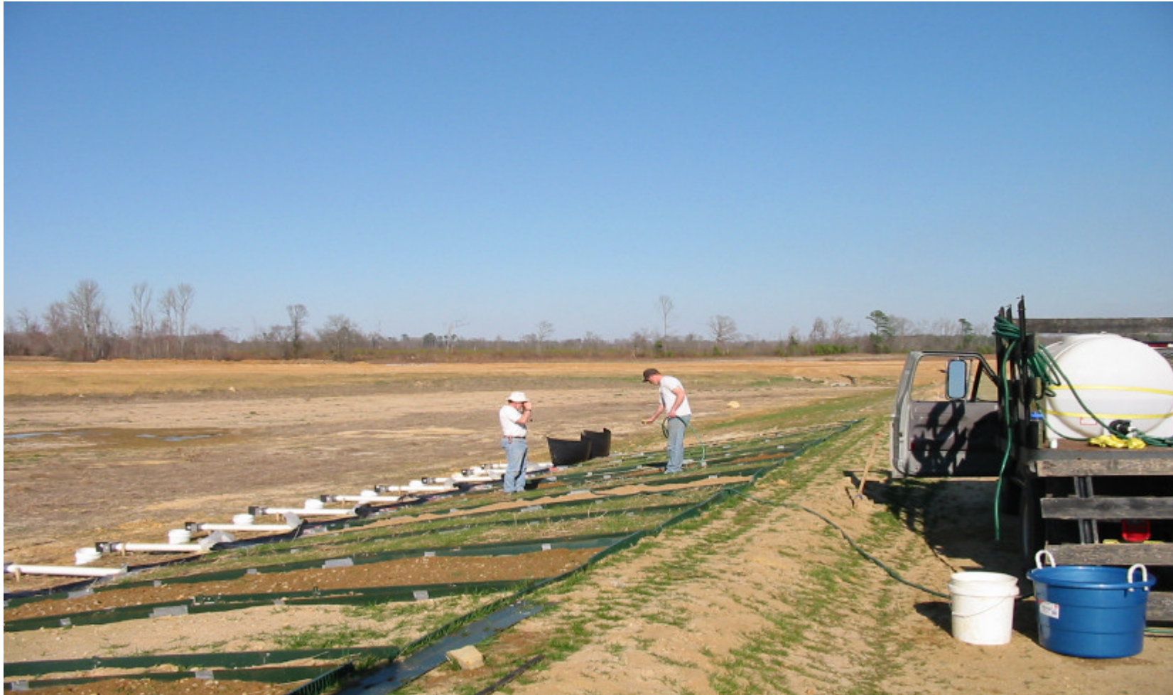
Figure 51. Applying PAM at highest rate (20 kg/ha) at the Fayetteville I-95 site.
